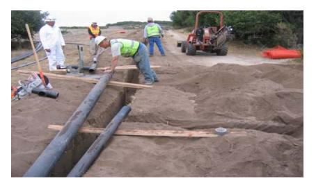
Photograph 1.1 – Trench excavation with ditch witch in background.
