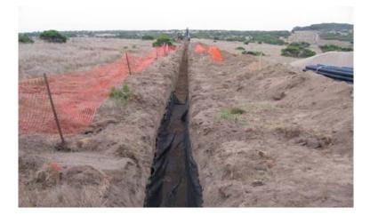
Photograph 1.3 – Excavation for injection trench.
