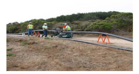
Photograph 1.2 – Laying out high density polyethylene pipe along the pipeline route.
