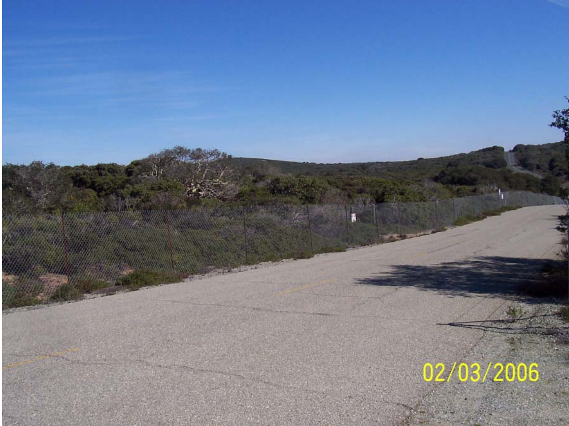
Picture 6: Heavy Vegetation within Primary Containment Line
