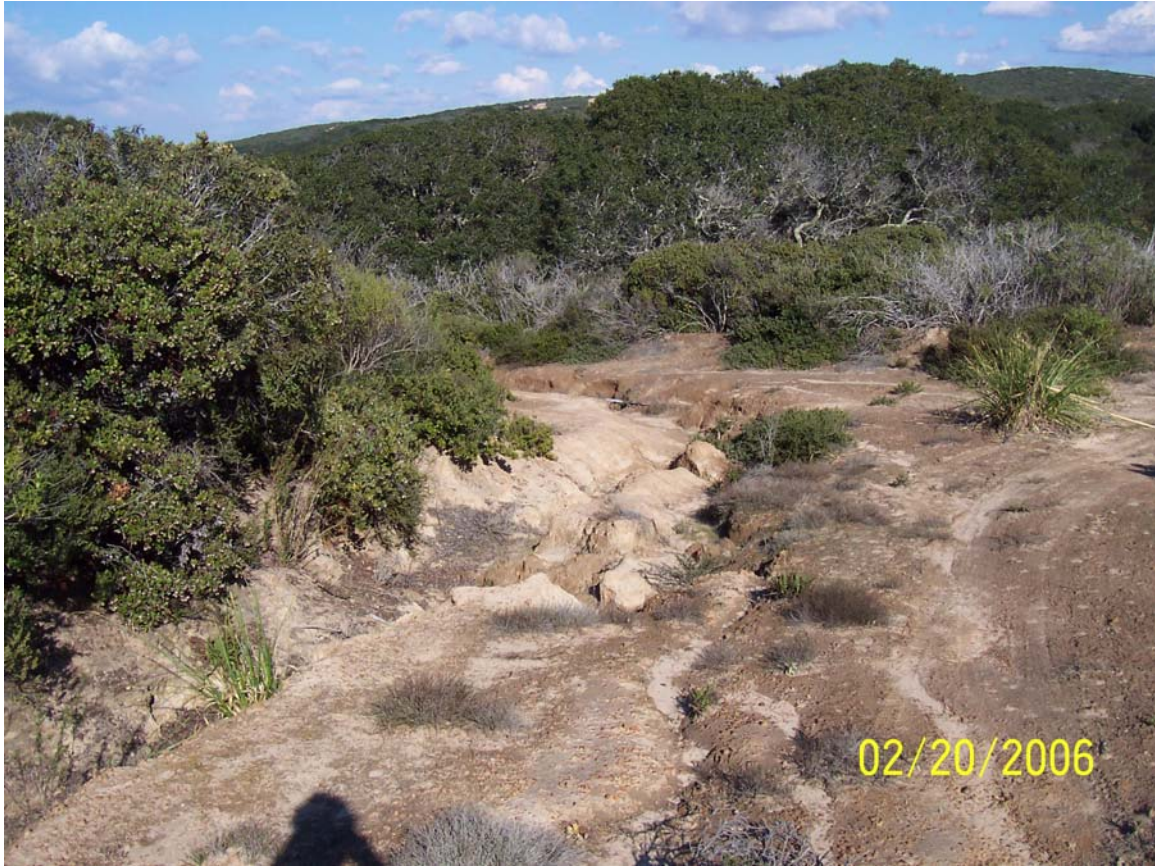
Picture 4: Rutted Section of Access Road
