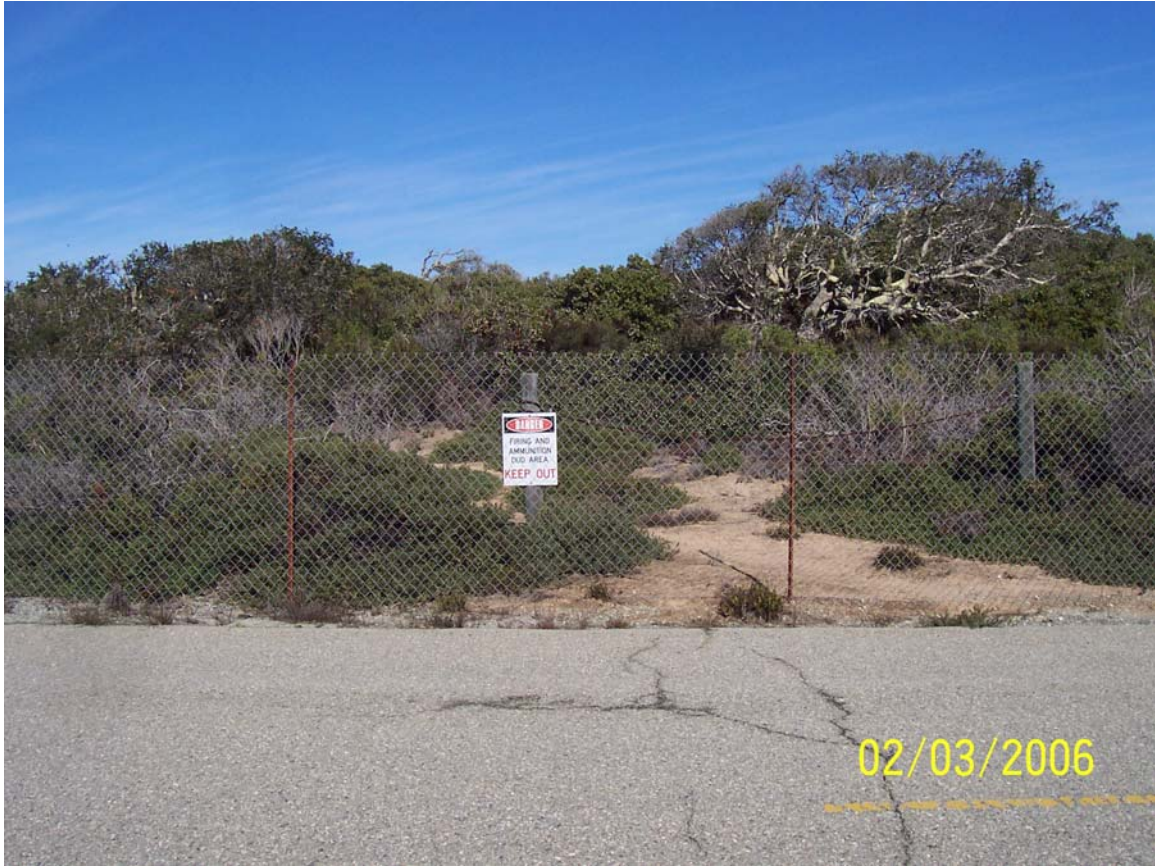
Picture 5: Heavy Vegetation within Primary Containment Line
