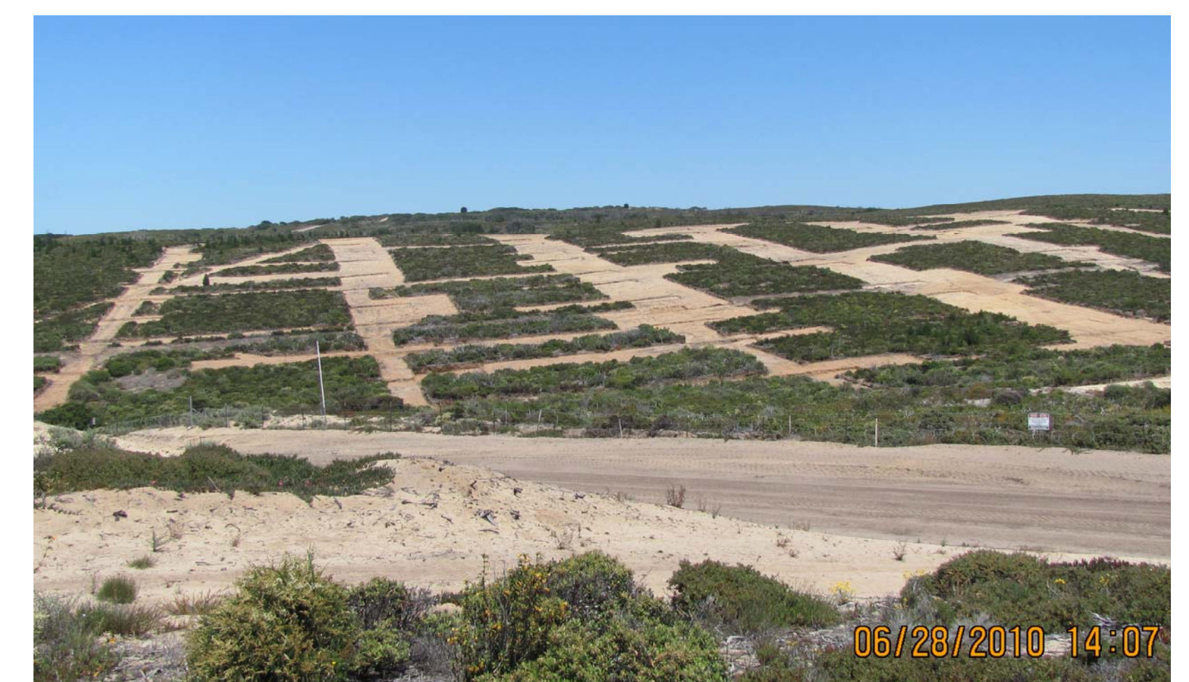
Typical range after remediation.
