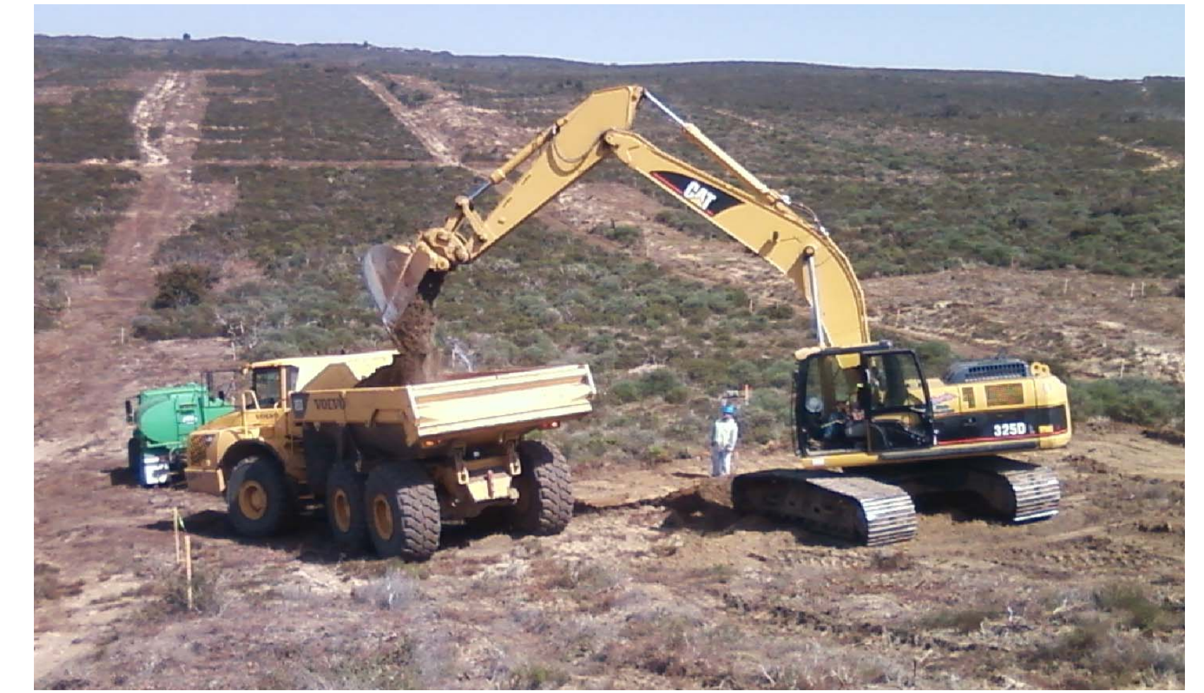
Excavator loads contaminated soil into off-road truck.
