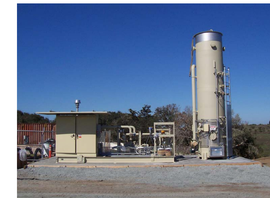
Landfill gas thermal treatment unit installed February 2006.
