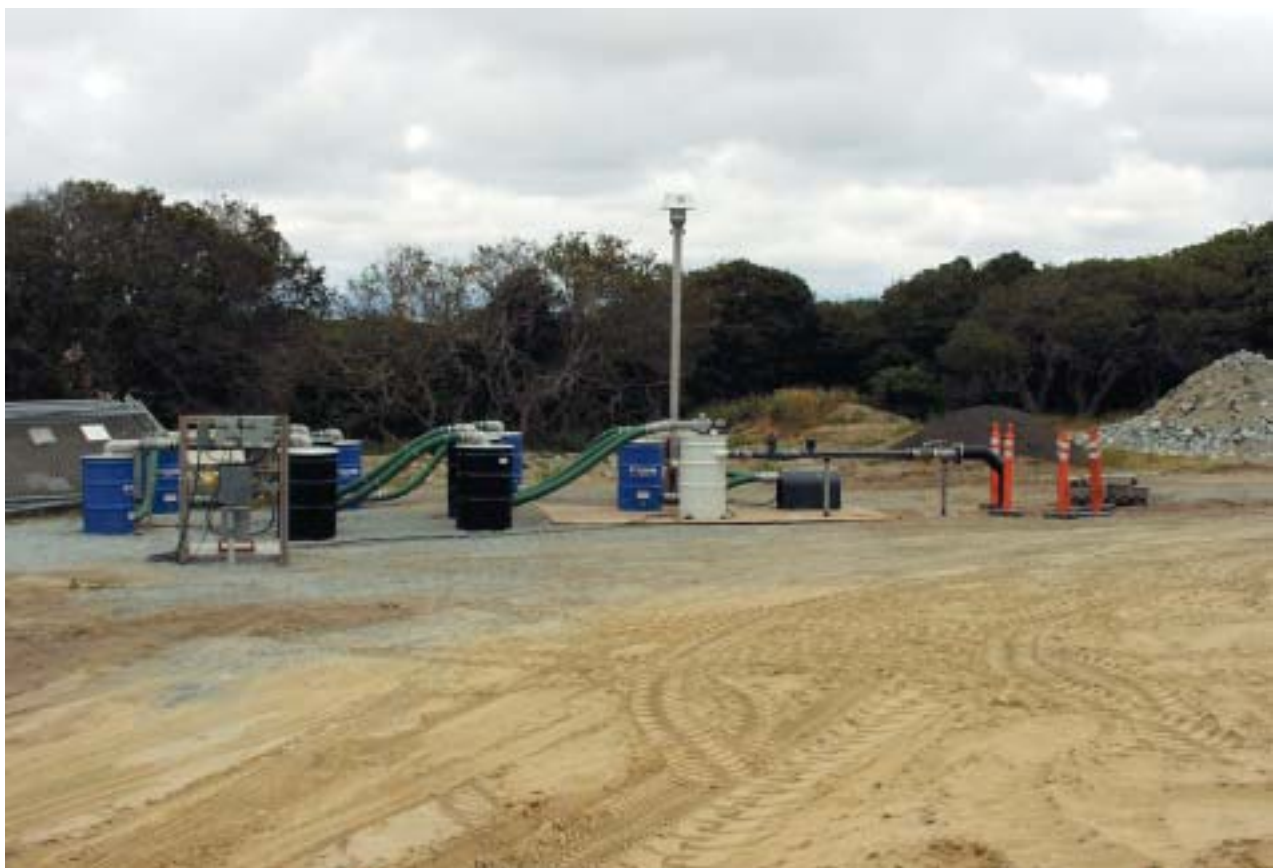
The Operable Unit 2 landfill gas collection and removal system designed and maintained by Shaw Environmental and Infrastructure, Inc.
