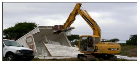
Structures like this wooden building in MOCO.2 were mechanically demolished.
