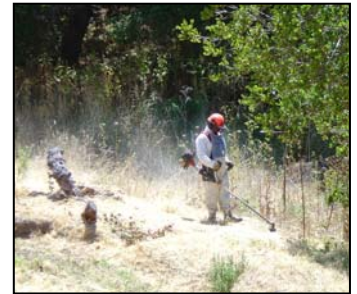
A worker cutting vegetation from the South Boundary Road fuel break with a string trimmer.
