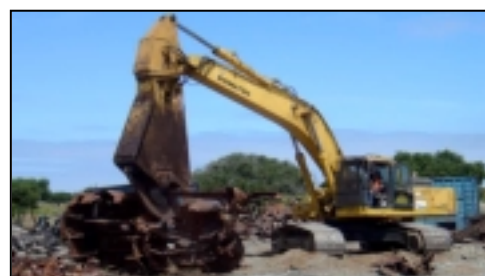
The mechanical shear cutting an old tank
