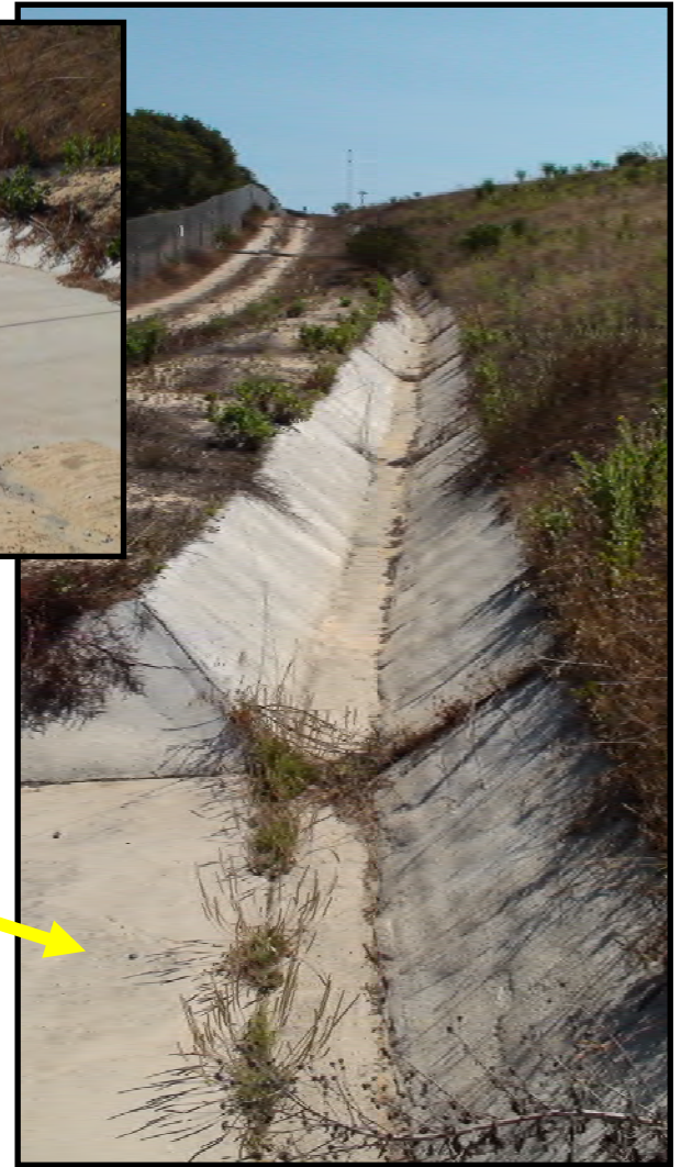
39. Area E eastern V-ditch facing south (August 3, 2020)
