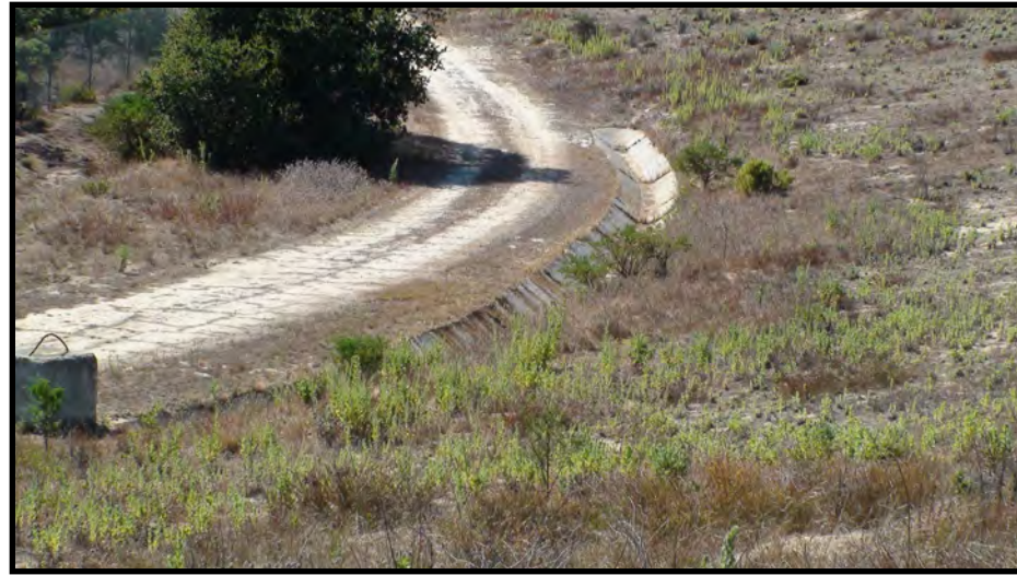
41. Area E central western V-ditch facing northwest (August 3, 2020)
