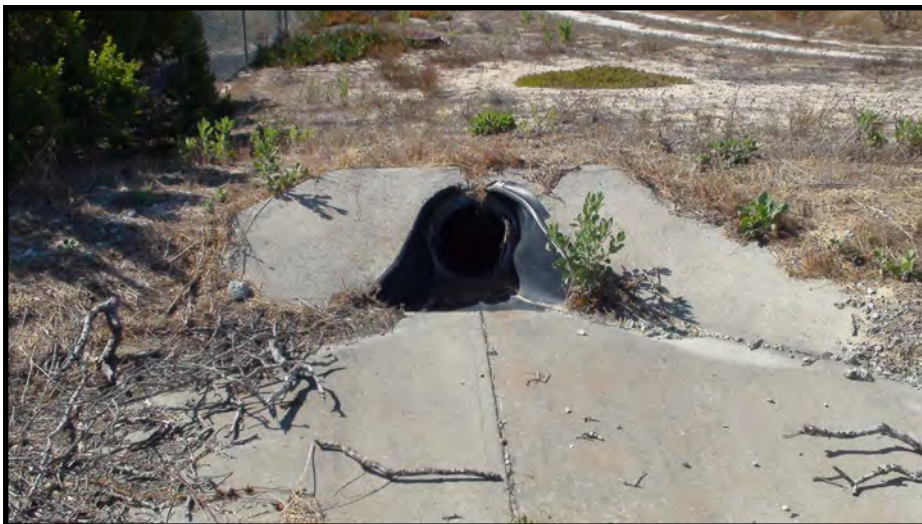
49. Drainage inlet from Engineer Equipment Road, southeast Area C (August 3, 2020)
