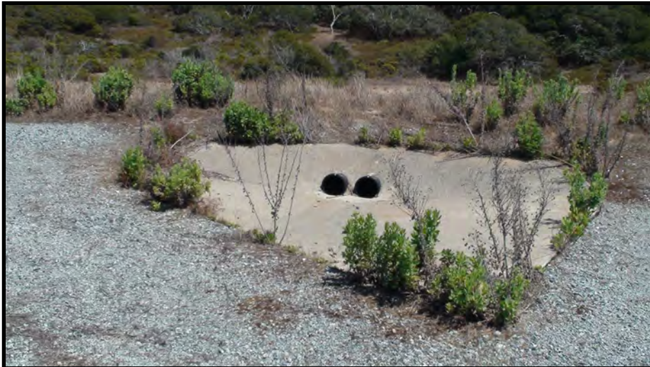
15. Downdrain inlet (two 8-inch pipes) on east side of Area D (August 3, 2020)
