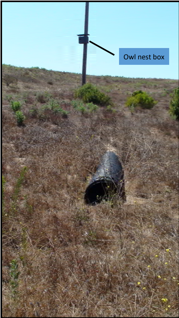
25. Northwest downdrain outlet (18-inch pipe), August 3, 2020
