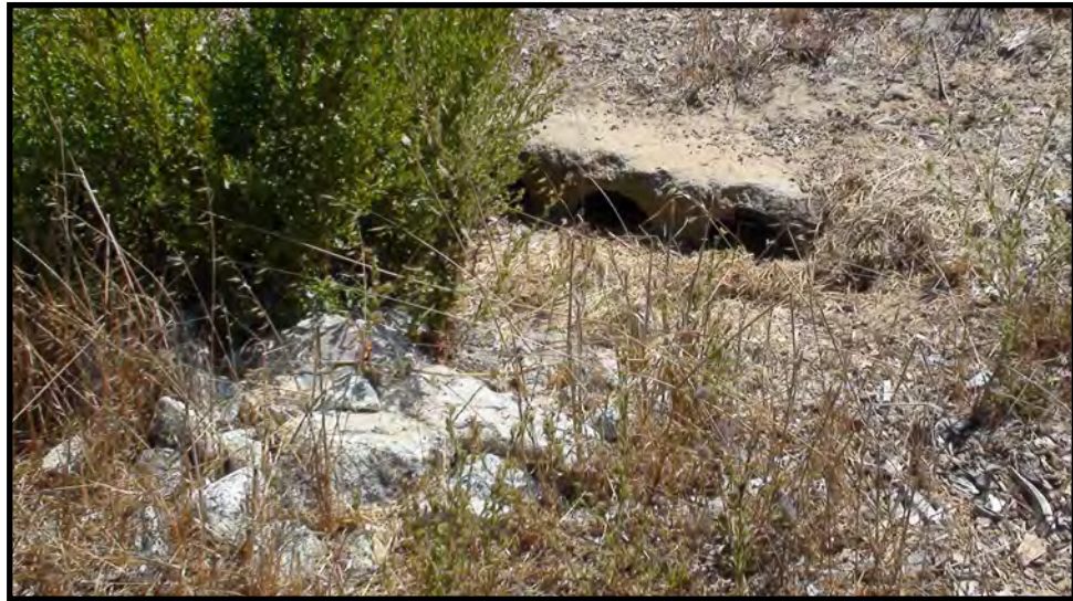
26. North central downdrain outlet (three 8-inch pipes), August 3, 2020
