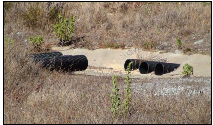
20. Northeast side downdrain transition apron (three 8-inch pipes), August 3, 2020
