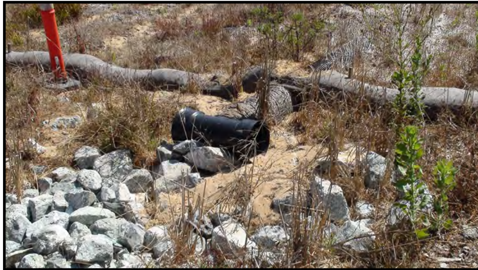
27. Subdrain downdrain outlet (one 8-inch pipe), August 3, 2020
