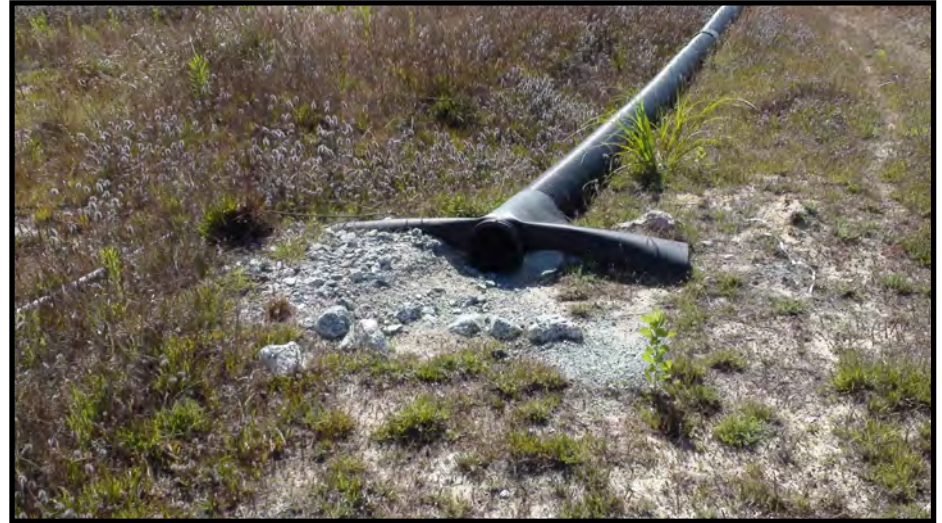
22. Phase 2 area temporary drainage inlet (August 3, 2020)
