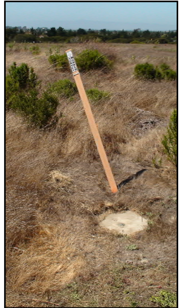
73. Area F Settlement Monitoring Plate SM-F2 (August 3, 2020)
