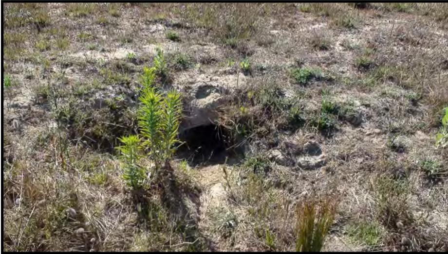
21. Phase 1 area brow ditch discharge point in Phase 2 area (August 3, 2020)
