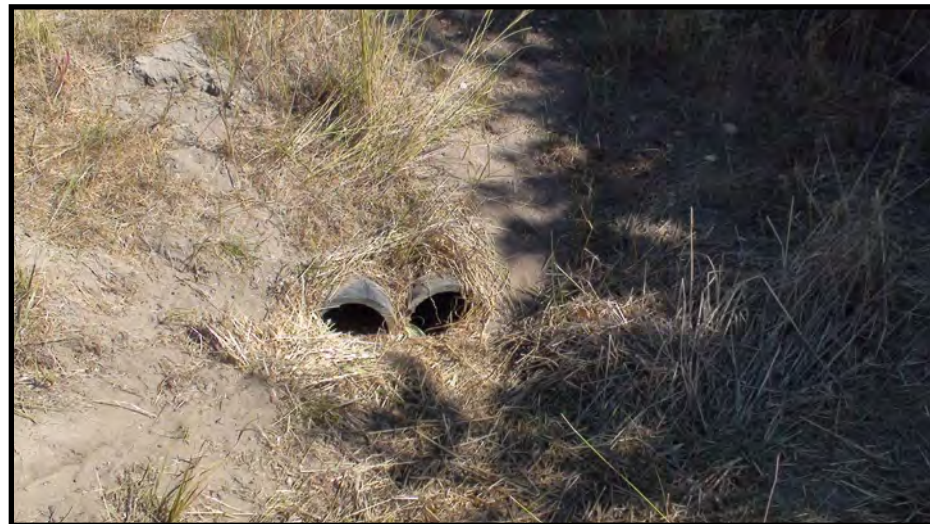
42. Area E southwestern/central western V-ditch discharge point (August 3, 2020), flows to infiltration basin
