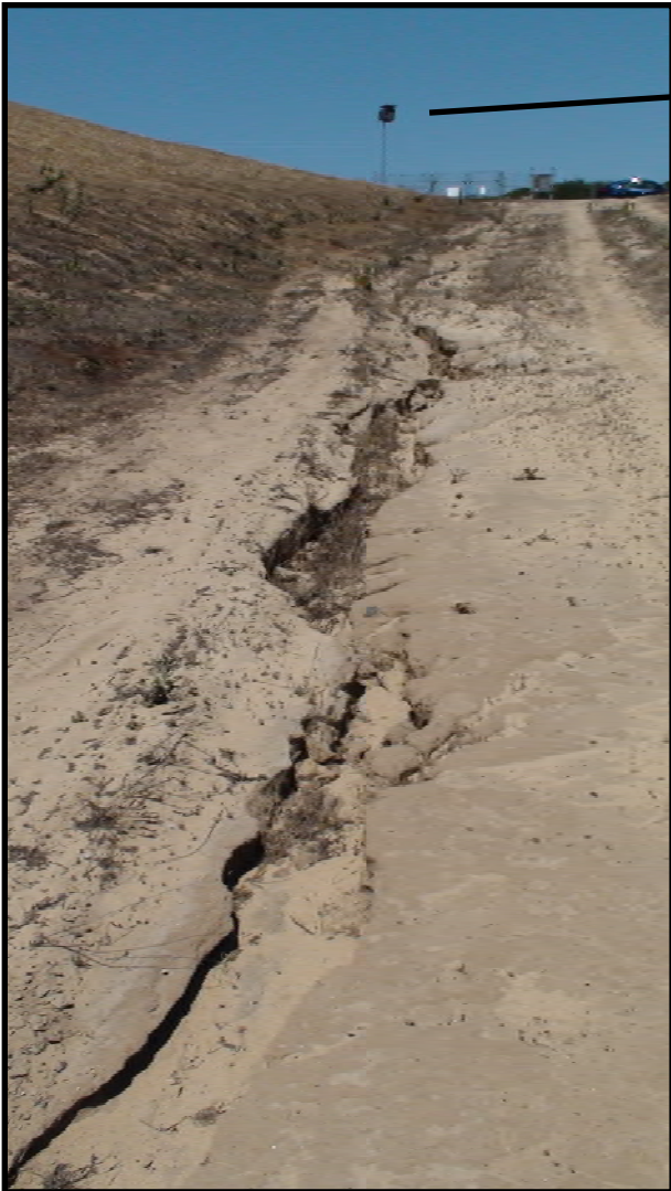
78. Perimeter service road erosion rills, east Area D facing northeast (August 3, 2020)
