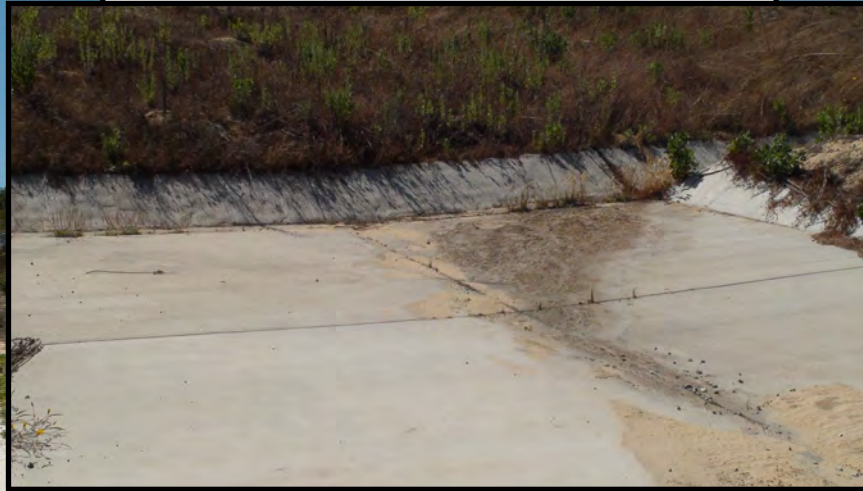
38. Area E eastern V-ditch concrete discharge apron facing west (August 3, 2020)
