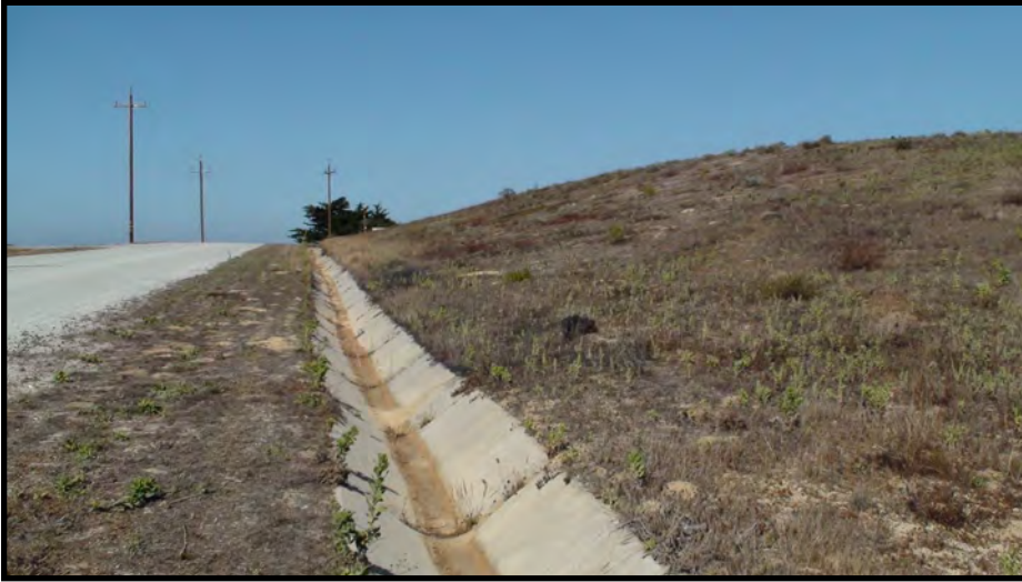
43. Area E northern V-ditch, facing northeast (August 3, 2020)
