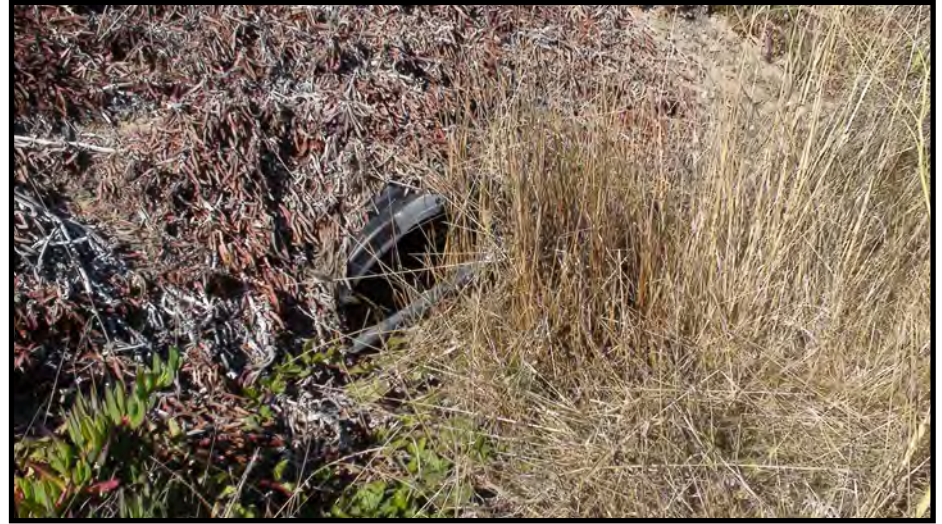
45. Area E northern V-ditch discharge point to infiltration basin (August 3, 2020)
