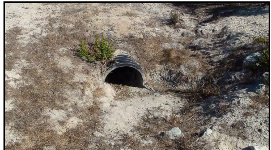
50. Drainage outlet, southwest Area C (August 3, 2020)
