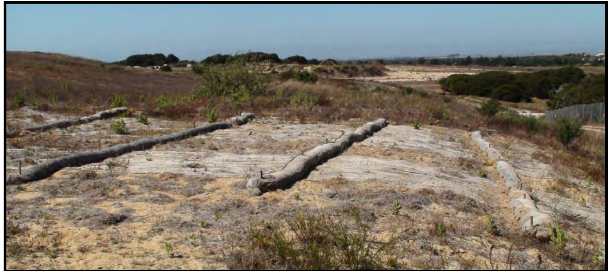
5. Area E east slope erosion repair facing north (August 3, 2020)
