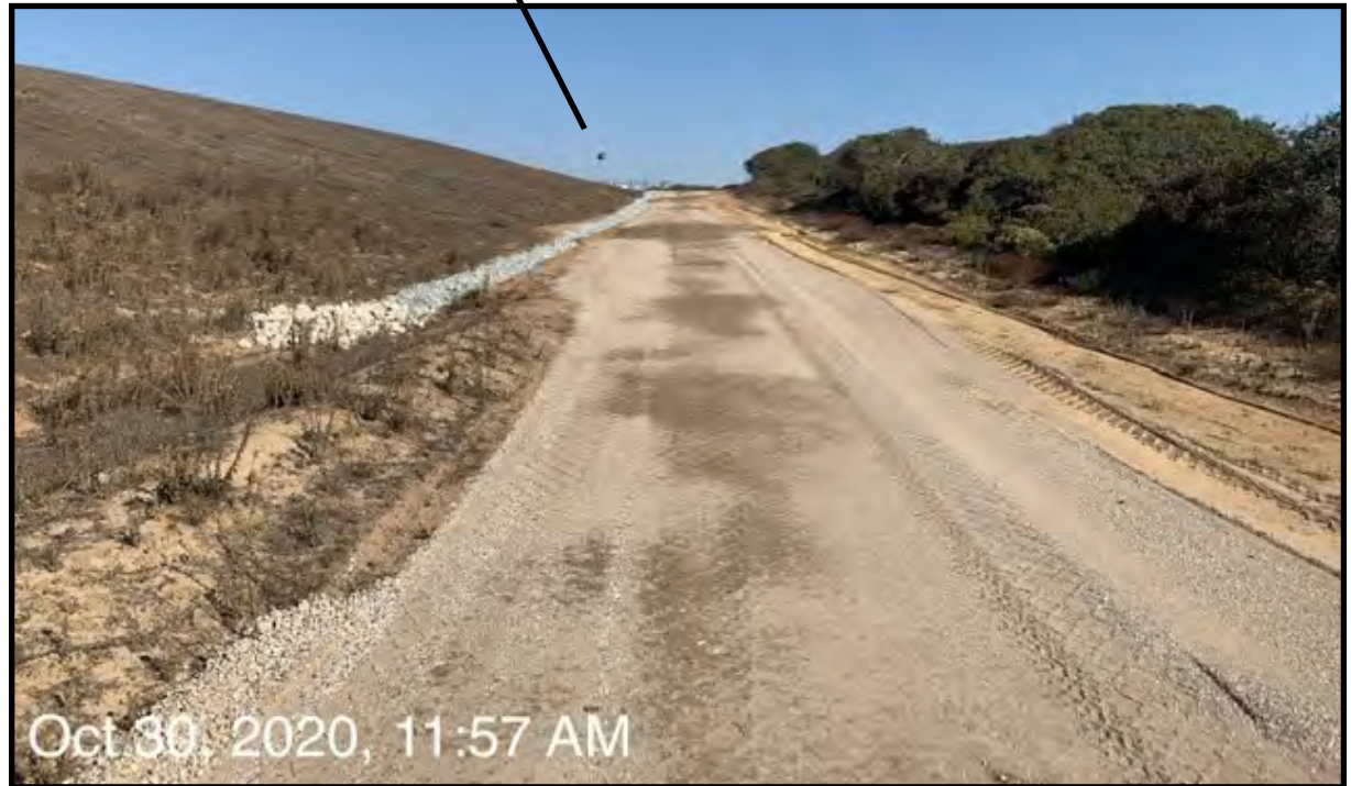
79. Perimeter service road repaired with rolling dips and rock-lined drainage swales, east Area D facing north-east (October 30, 2020)
