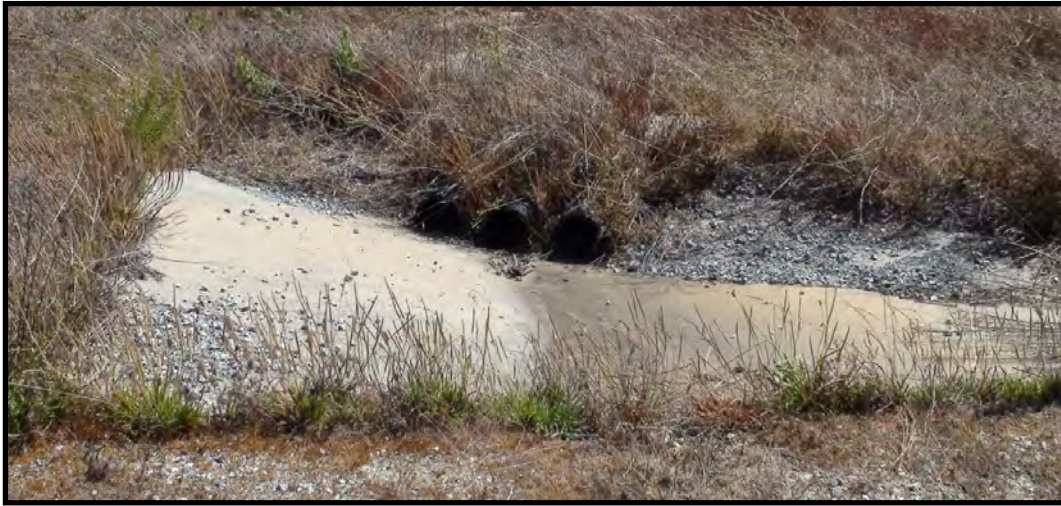
28. Southeast downdrain inlet (three 8-inch pipes), August 3, 2020
