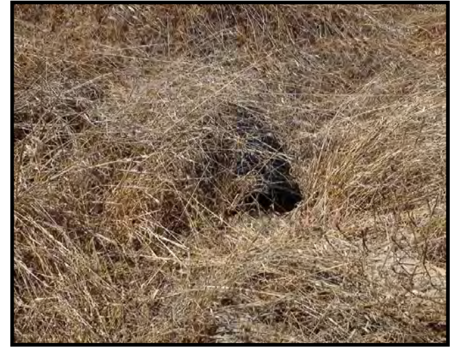
29. Southeast downdrain outlet (three 8-inch pipes), August 3, 2020
