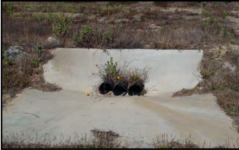
17. Southeast side downdrain catch basin (three 8-inch pipes), August 3, 2020
