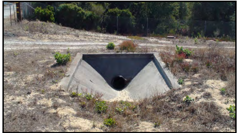
48. Drainage inlet from southeast Area C swale (August 3, 2020)
