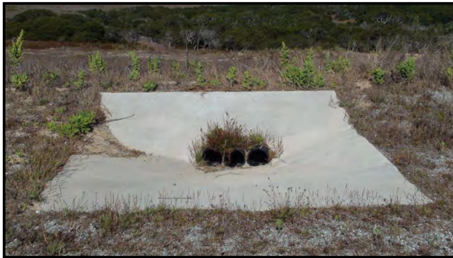
19. Northeast side downdrain catch basin (three 8-inch pipes), August 3, 2020
