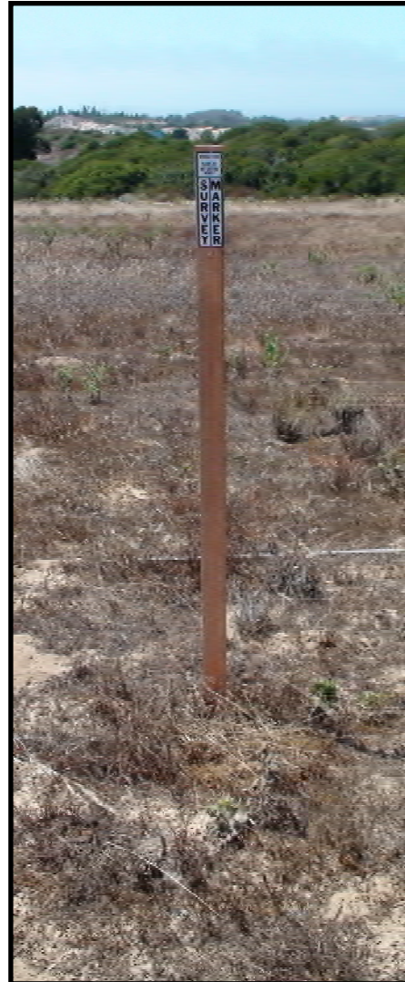
65. Area D Settlement Monitoring Plate SM-D1 (August 3, 2020)
