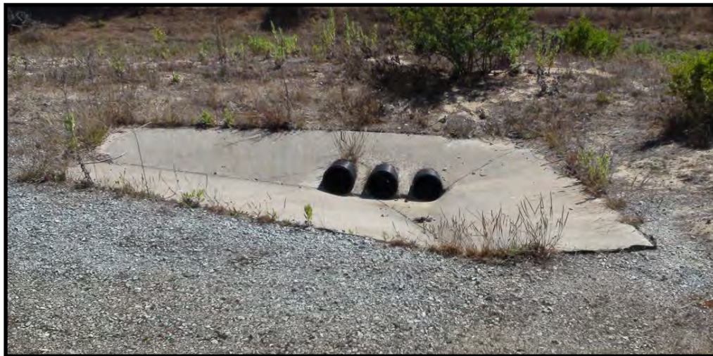
30. Southwest downdrain inlet (three 8-inch pipes), August 3, 2020
