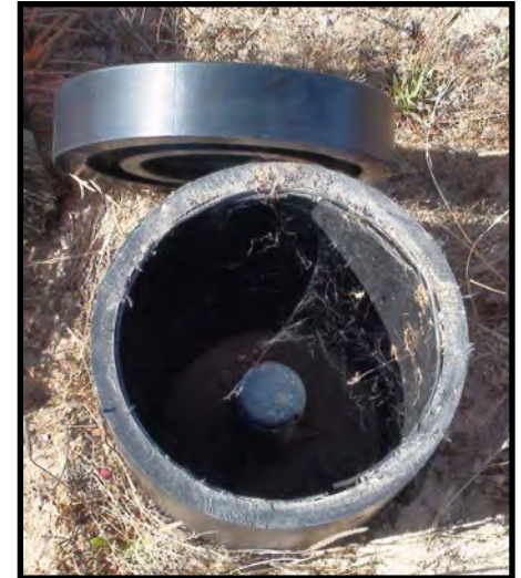
70. Area E Settlement Monitoring Plate SM-E4 (August 3, 2020)
