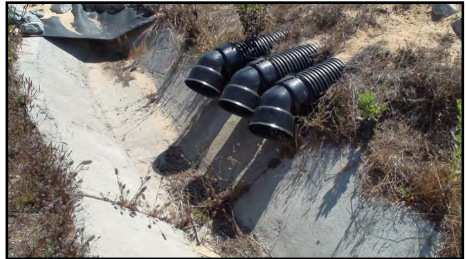
18. Southeast side downdrain outlet (three 8-inch pipes), August 3, 2020
