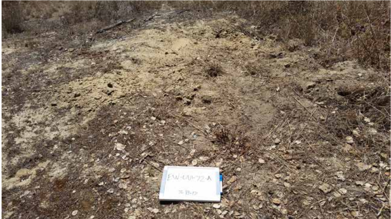
Site condition after completing destruction and demobilization at well EW-OU1-72-A
