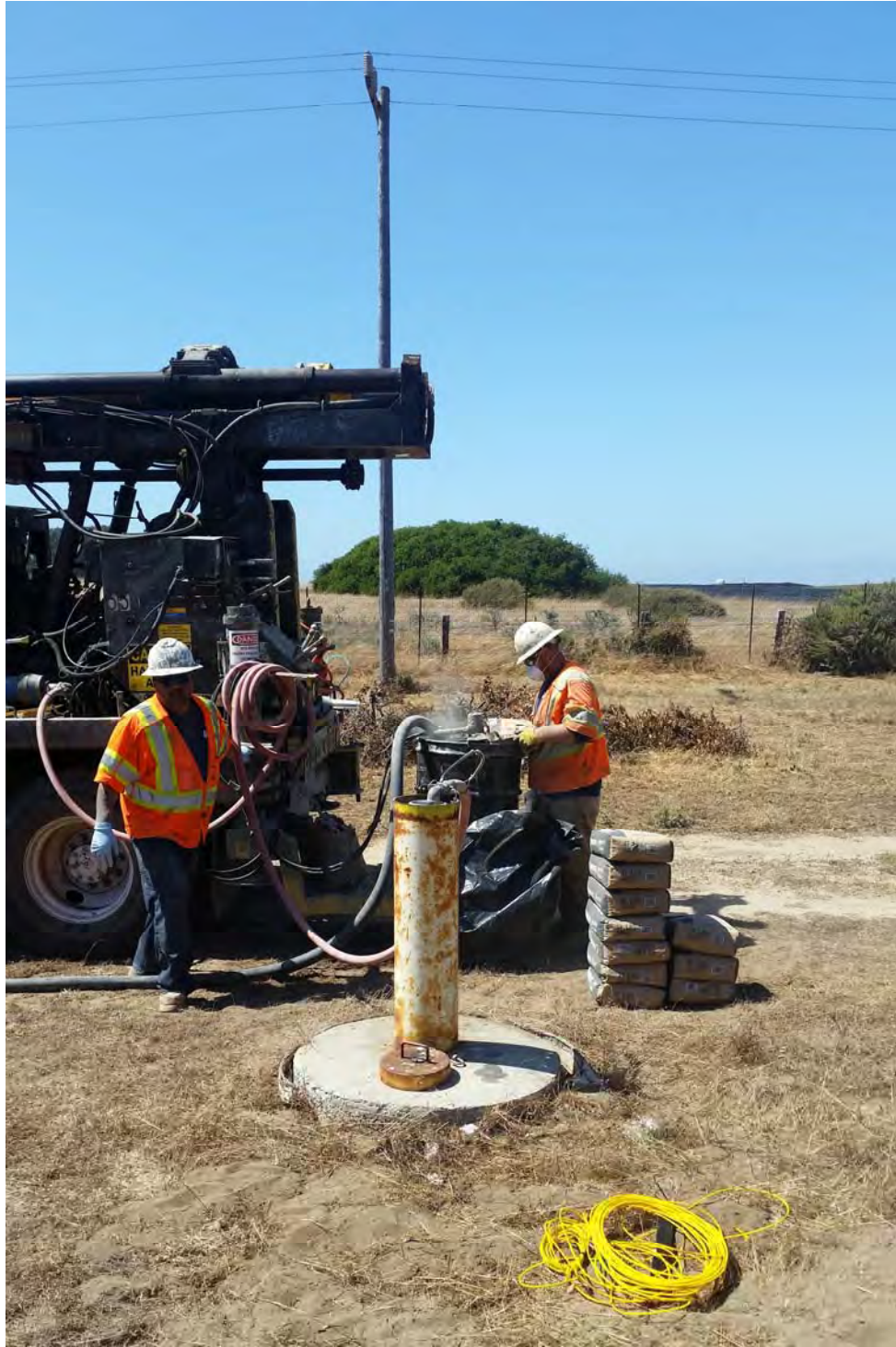
Mixing and pumping grout to seal well on northwest boundary 20170711_152623
