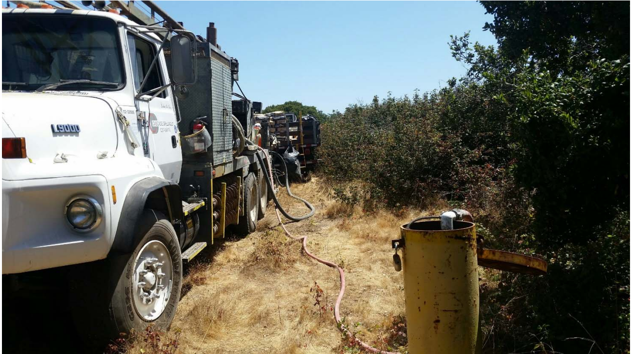
Photo 01 –Pressure grouting EW-OU1-52-A.
