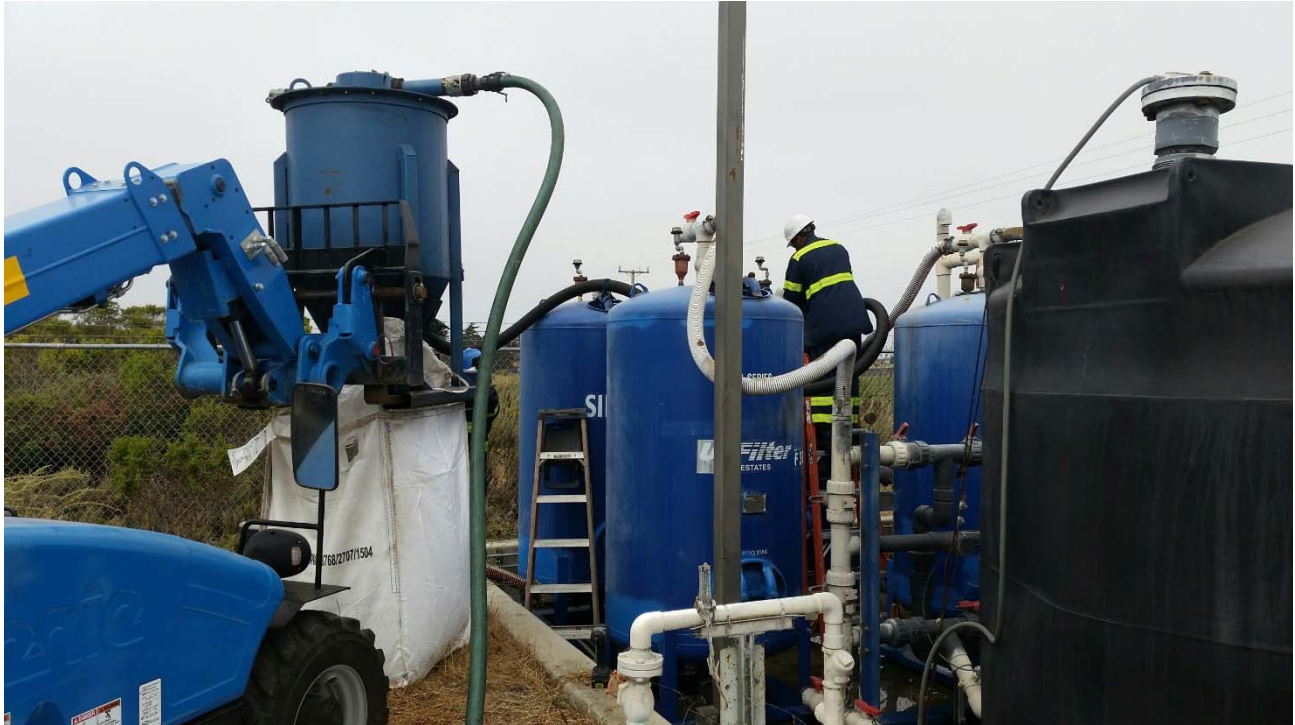
Photo 02 – Removing GAC from vessels.
