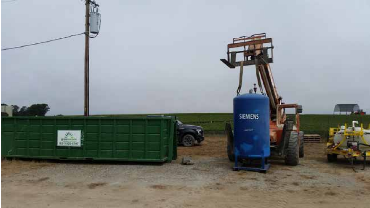
First carbon vessel removed and staged for transport
