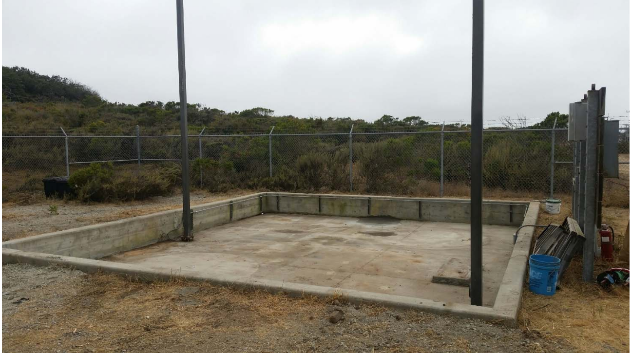
Photo 03 – NWTs decommissioning complete.
