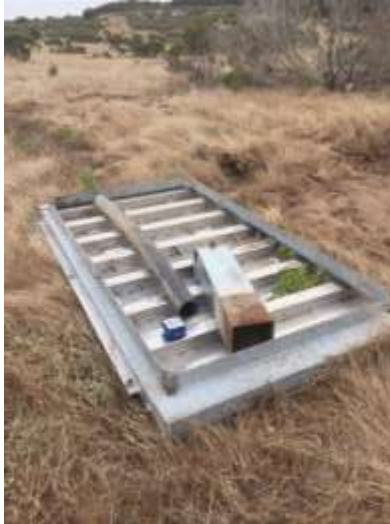
Photograph 6 – FONG infiltration trench vault lid.
