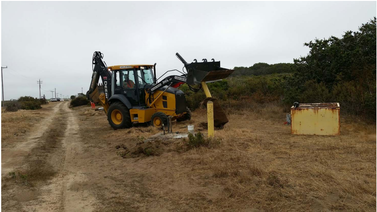
Photo 01 – Removing bollards and surface completion.
