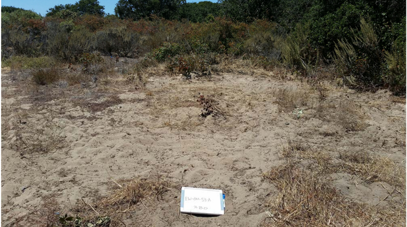
Photo 02 – Well destruction and restoration complete at EW-OU1-53-A.
