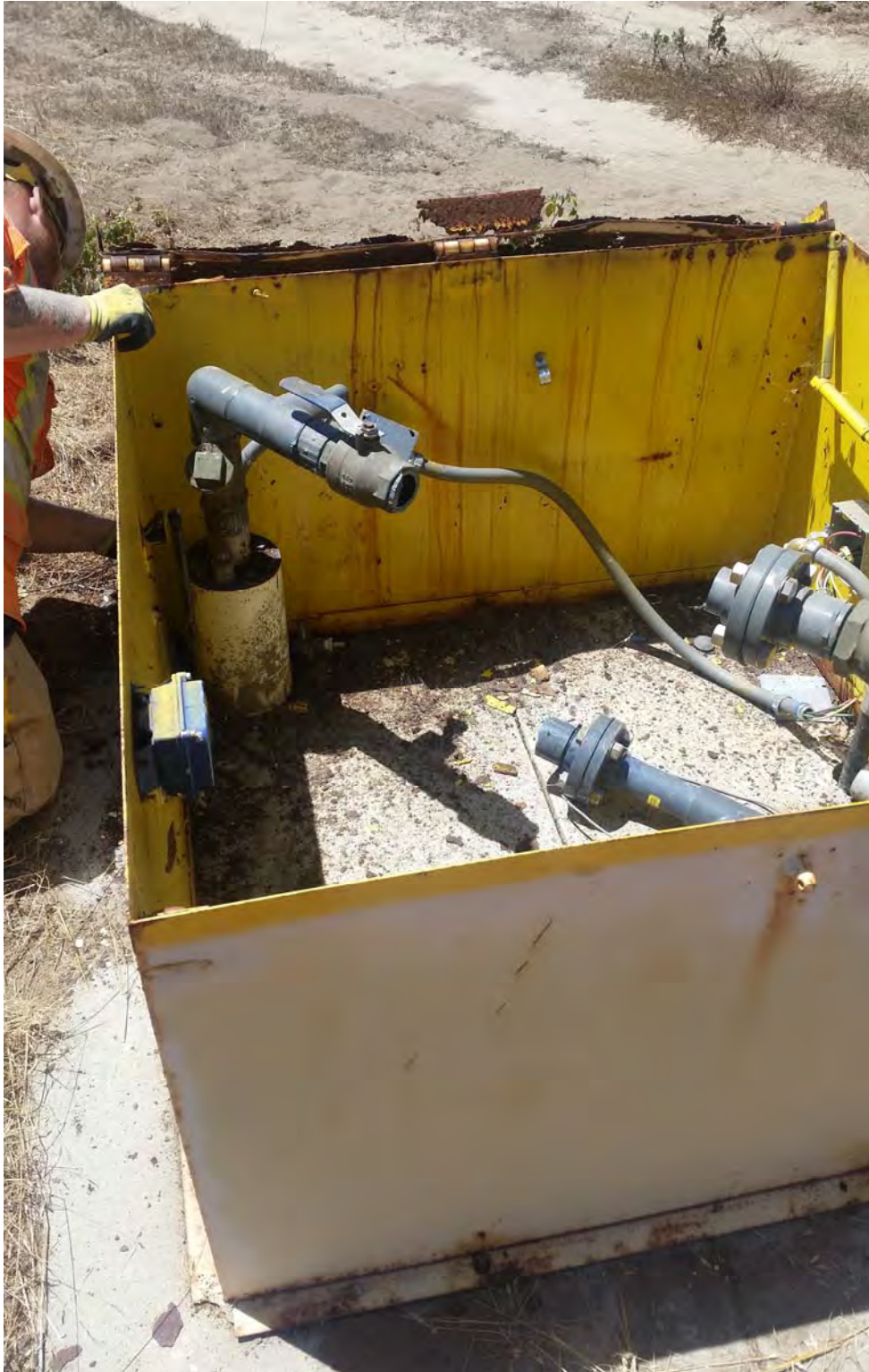
Removing well housing and pipe on boundary well
