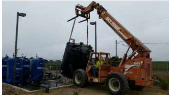
Photograph 4 – Removing holding tank at NWTS. Equipment shown: SkyTrak 10054 telescopic forklift.
