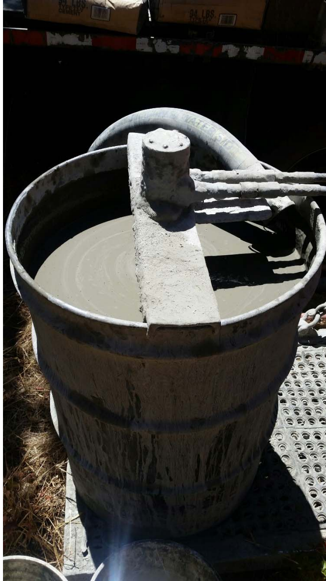
Photo 03 – Mixing grout.
