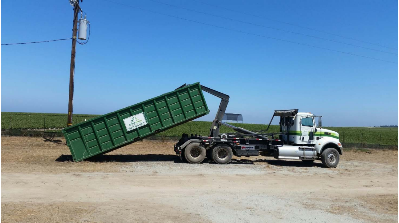
Photo 01 – Roll off bin of construction debris picked up for disposal.
