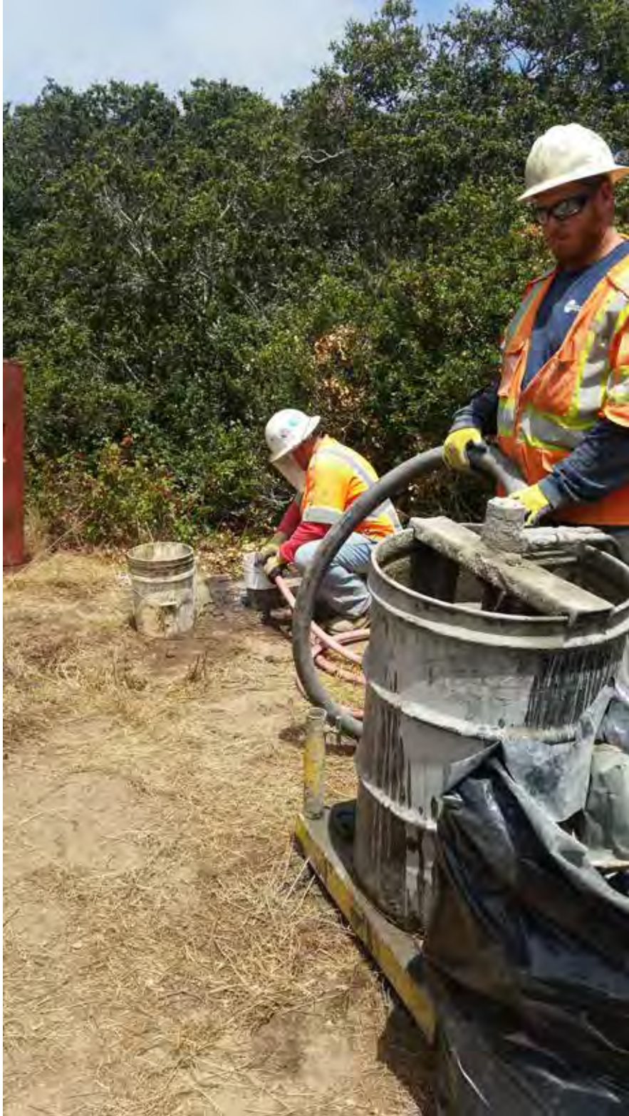
Mixing and pumping grout to seal well in habitat area 20170714_132221
