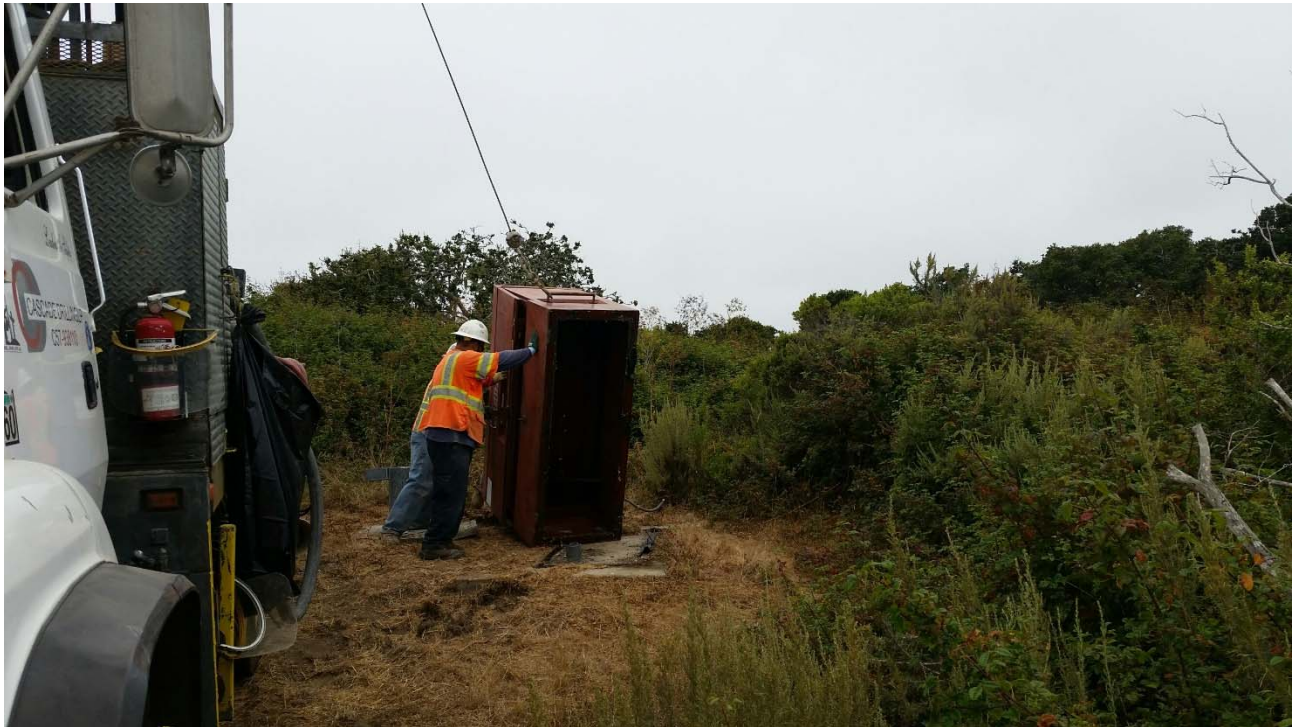
Photo 01 – Removing protective housing at MW-OU1-46-AD.
