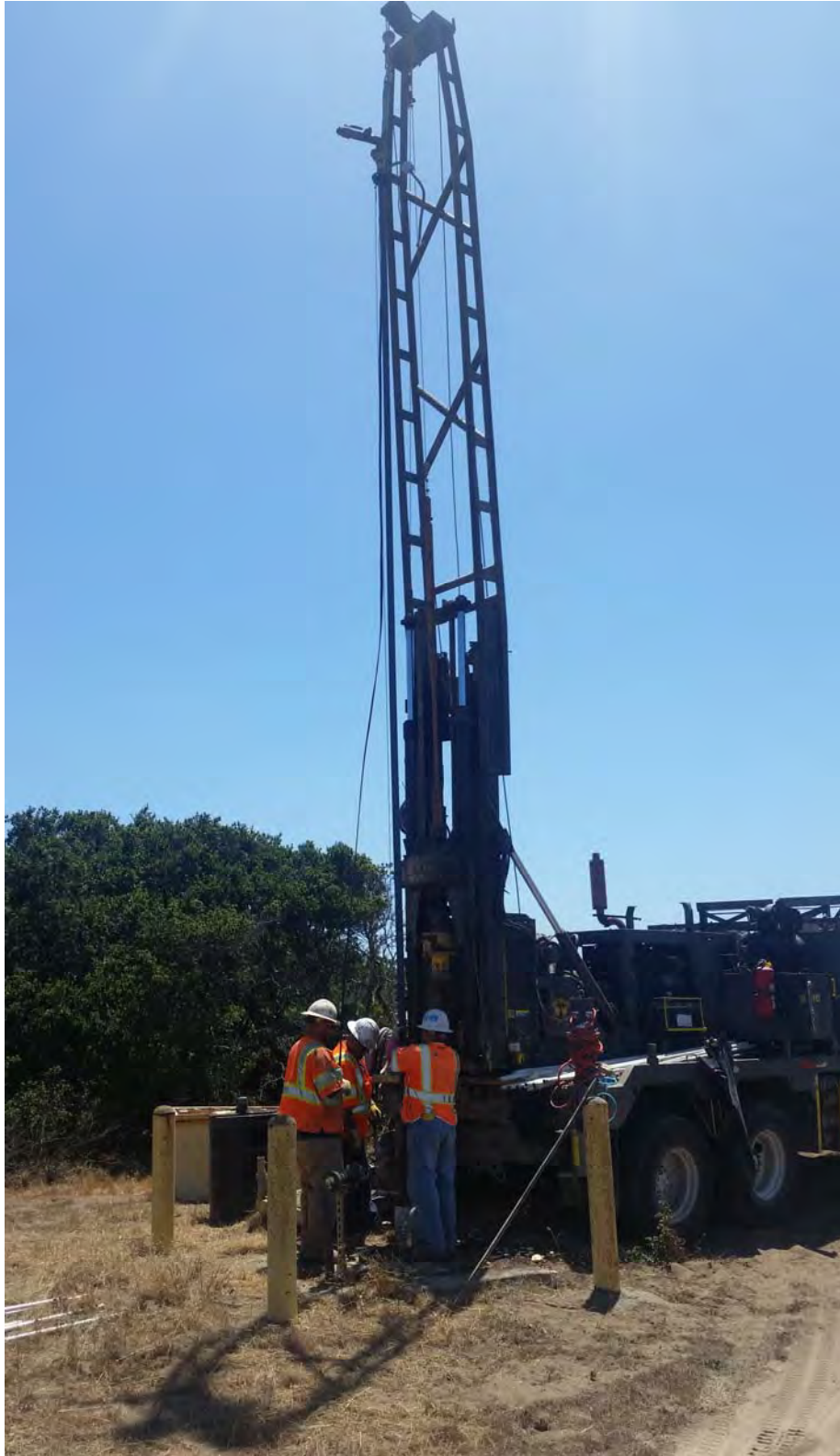
Removing pump from extraction well
