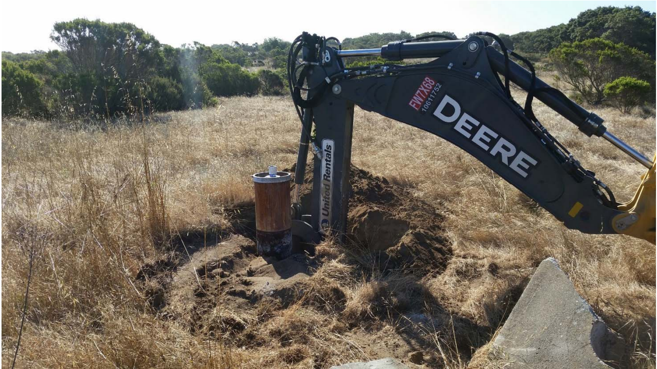
Photo 01 – Excavating to 5 ft bgs to remove casing at MW-OU1-27-A.
