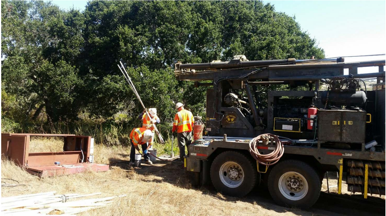
Photo 02 – Pressure grouting.
