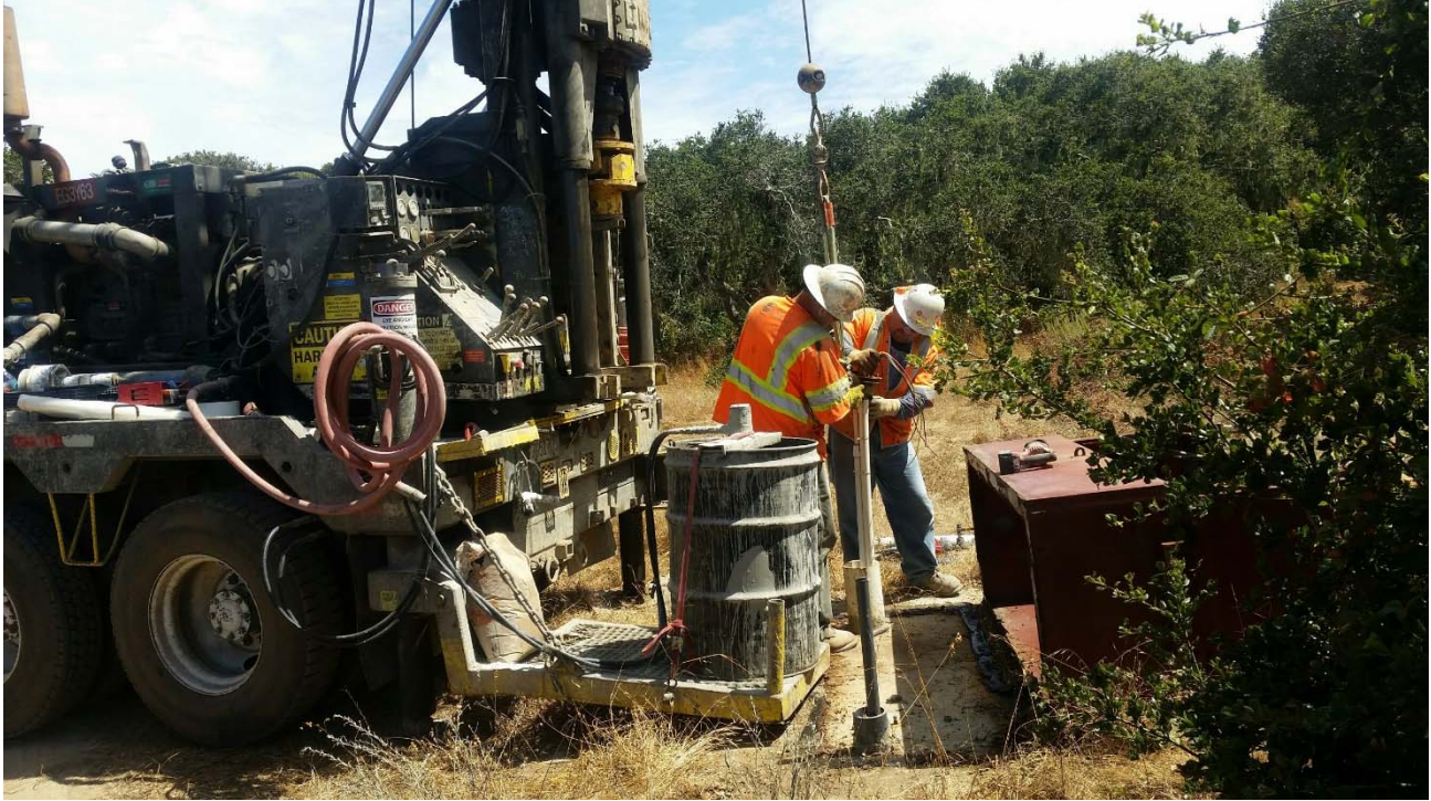
Photo 03 – Removing extraction pump.
