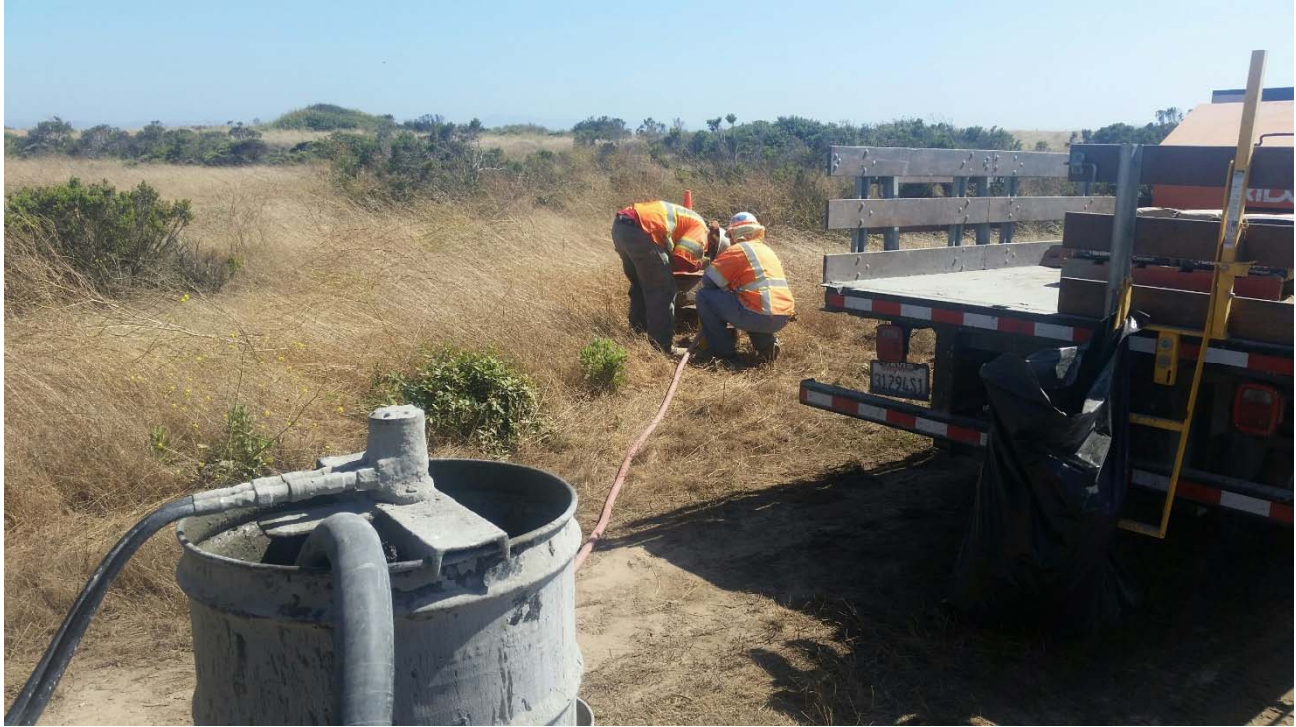
Photo 03 – Grouting MW-B-02-A.
