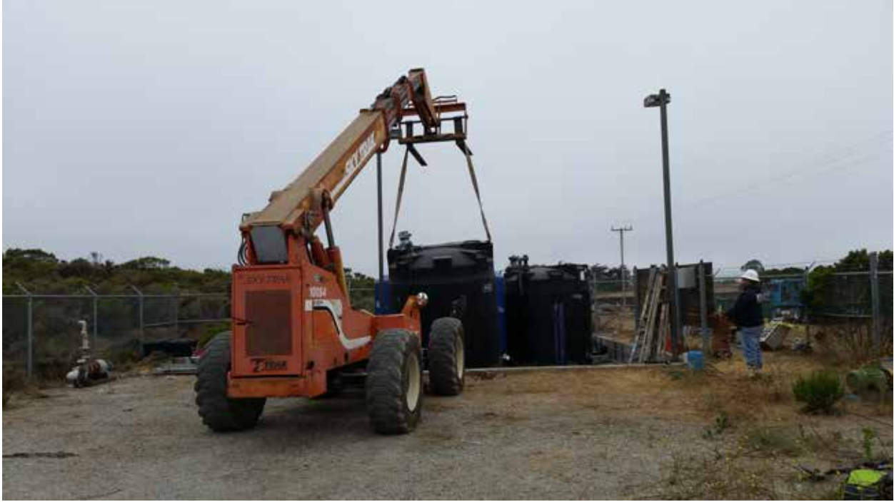
Removing treated water holding tank from NWTs containment basin
