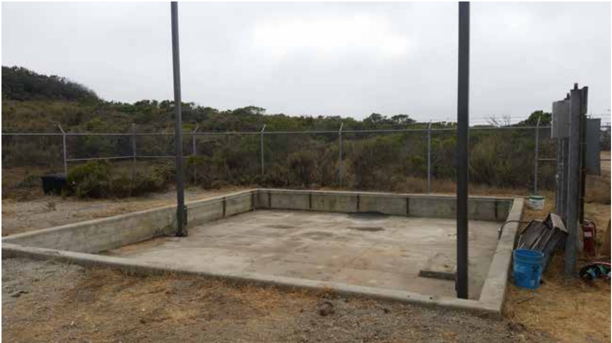
NWTS containment basin after decommissioning
