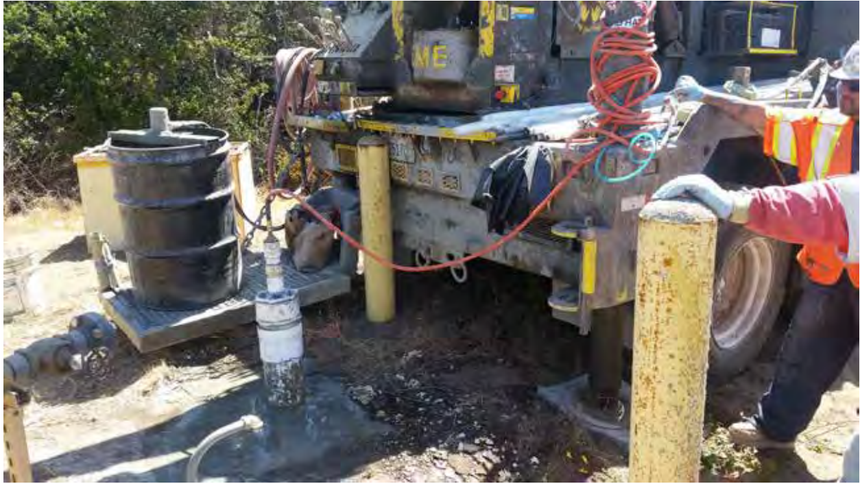
Well sealing operation equipment setup
