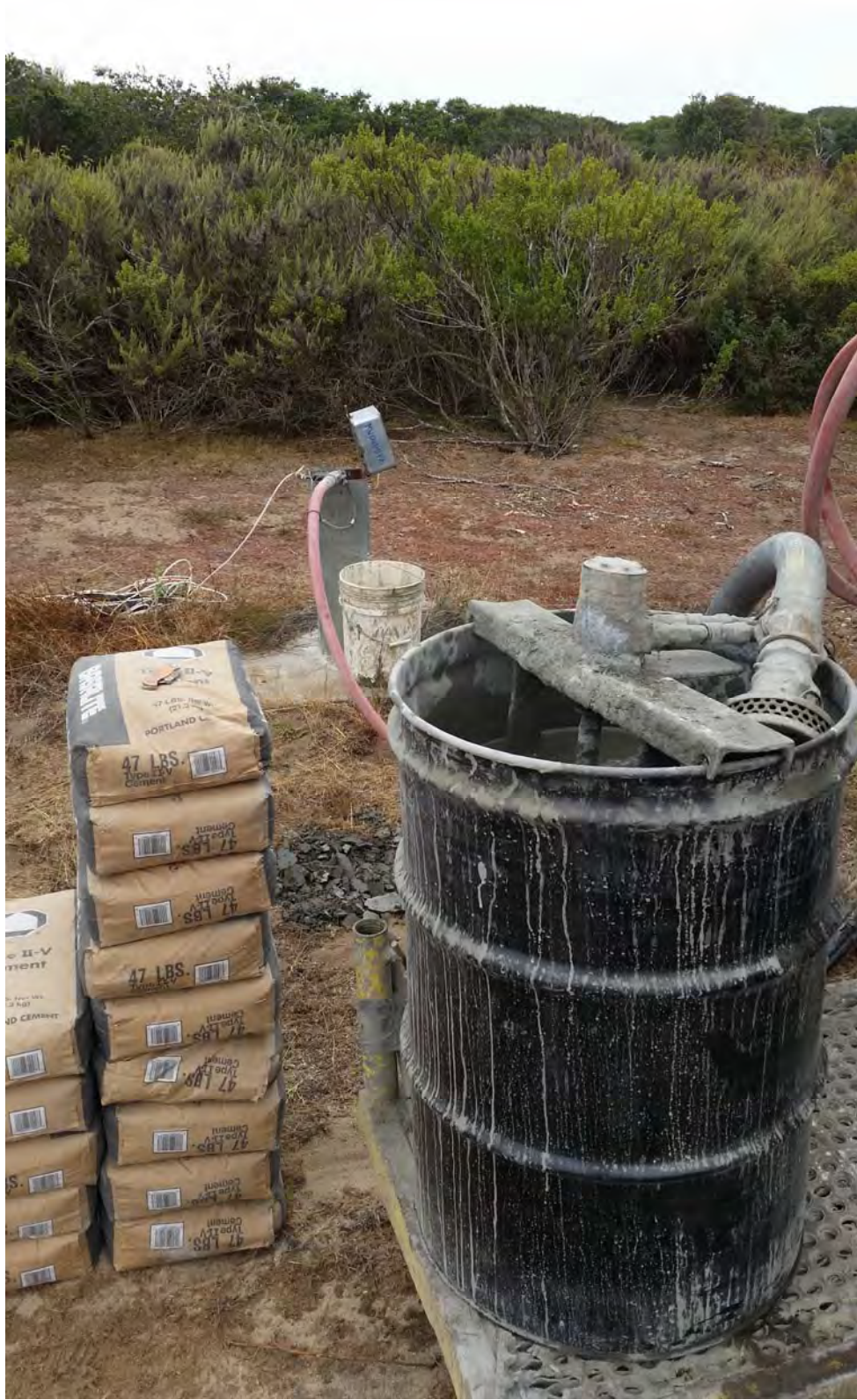
Grout mixing setup
