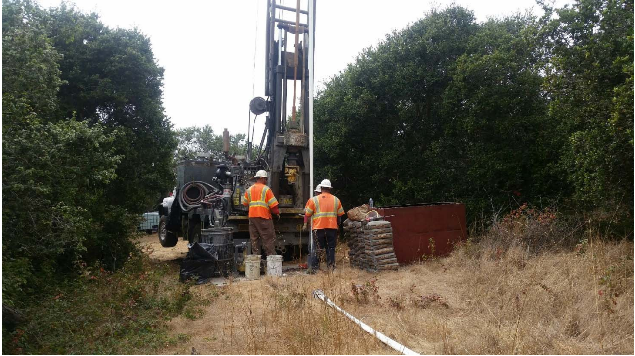
Photo 03 – Pulling injection pipe at IW-OU1-73-A.
