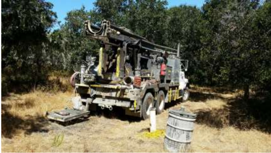
Photograph 1 – Setting up to pressure grout. Equipment shown: CME 75 drill rig.
