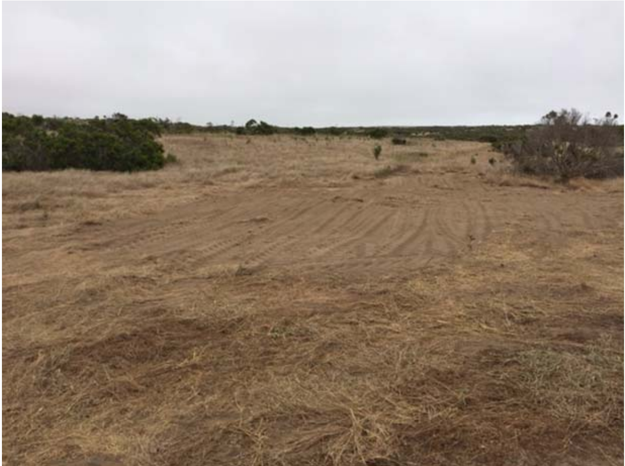
Photo 04 – Grassland Surface After Treated Water Infiltration Vault Removed
