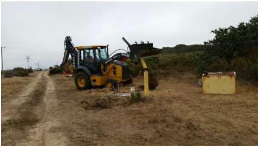
Photograph 2 – Removing bollards and surface completion. Equipment shown: John Deere 310L Backhoe.
