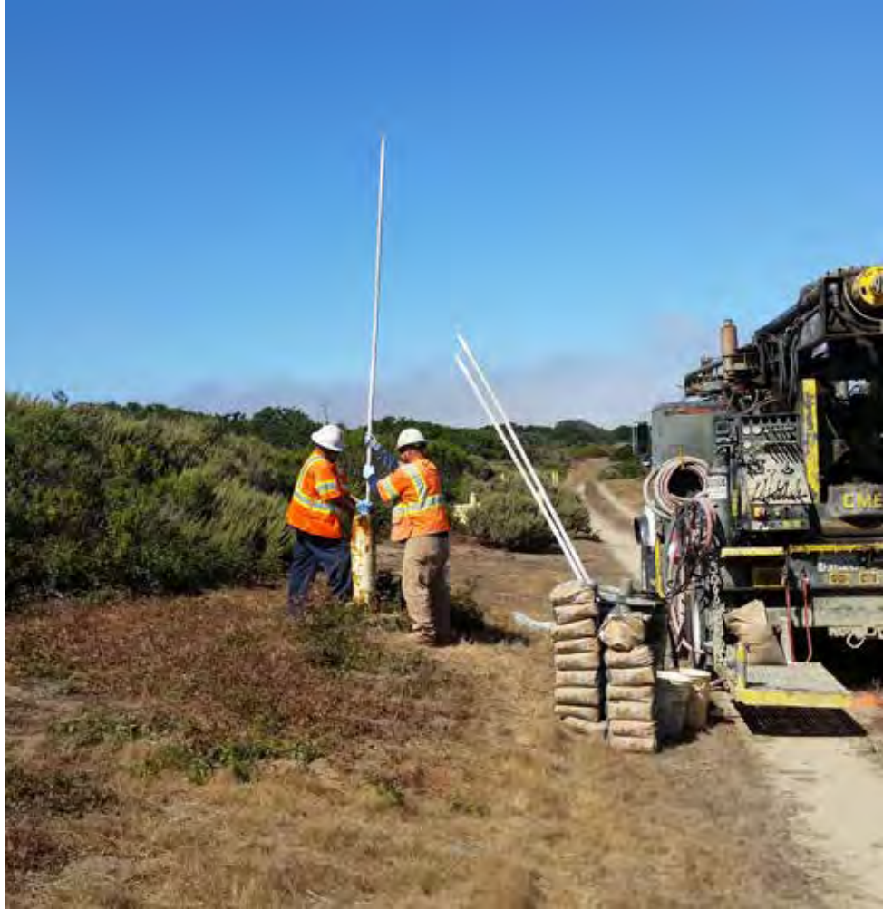
Setting tremie pipe before grouting
