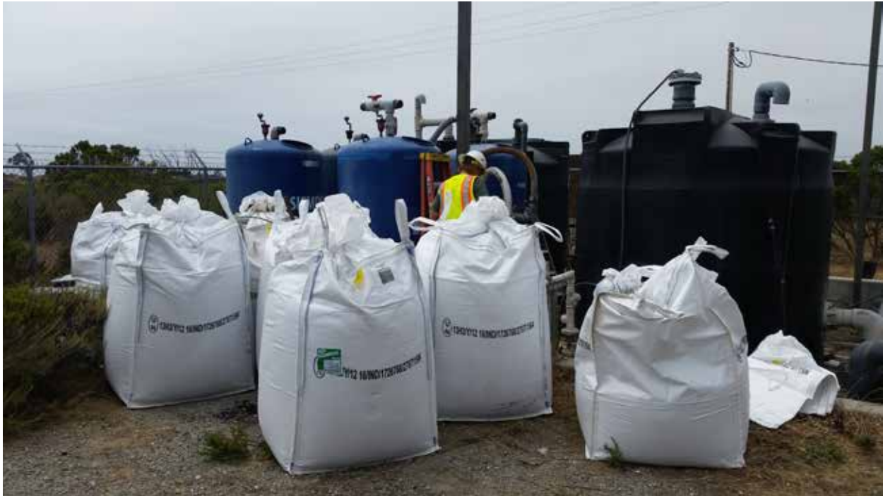
Carbon from NWTs in bags staged for transport to regeneration facility
