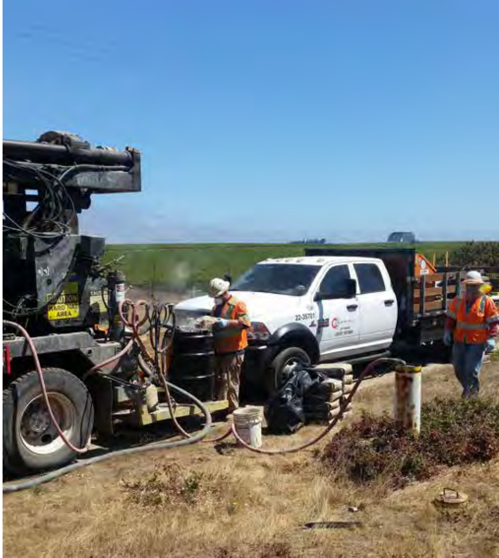
Well sealing in progress
