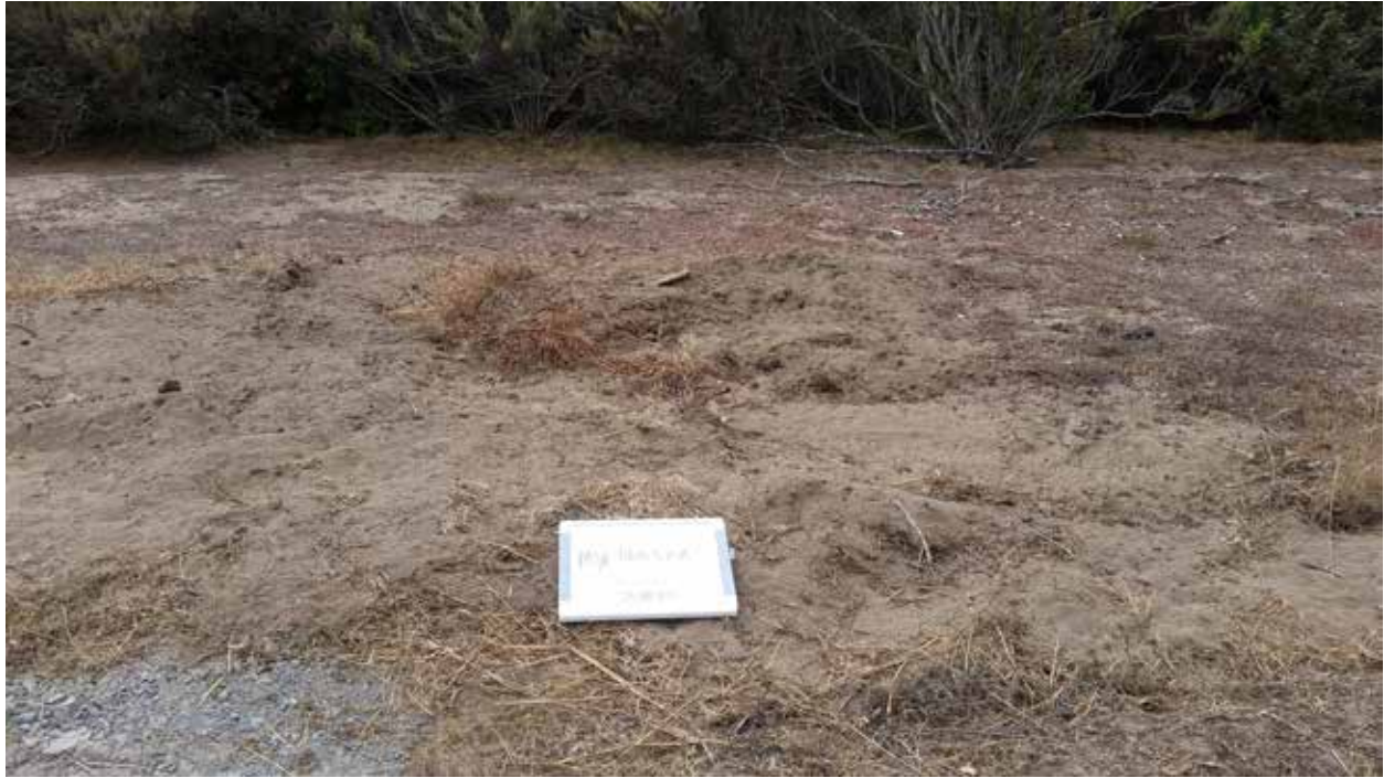
Site condition after completing destruction and demobilization at well MW-OU1-57-A 20170718_110656
