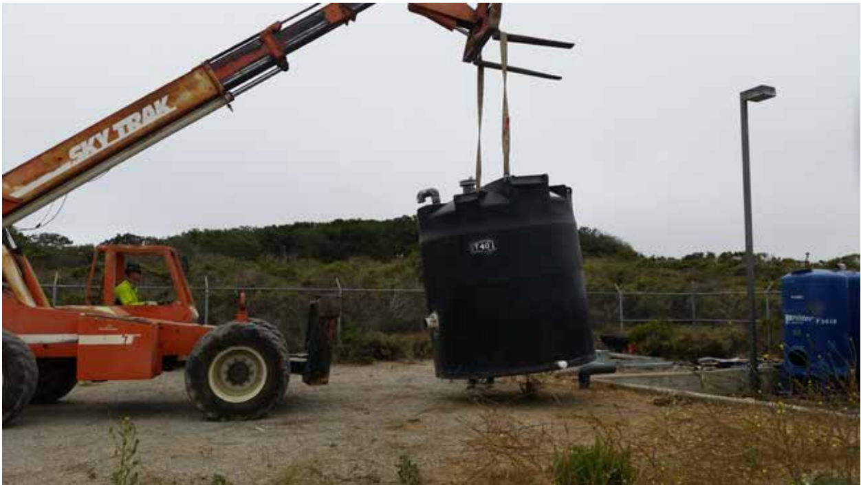
Transporting treated water holding tank from NWTs
