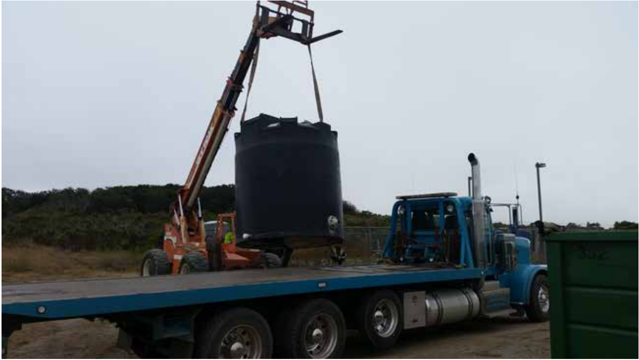
Loading treated water holding tank for transport
