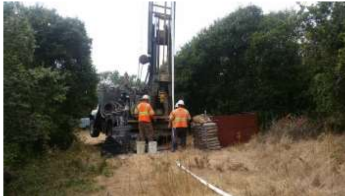
Photograph 3 – Pulling injection pipe at IW-OU1-73-A. Equipment shown: CME 75 drill rig.
