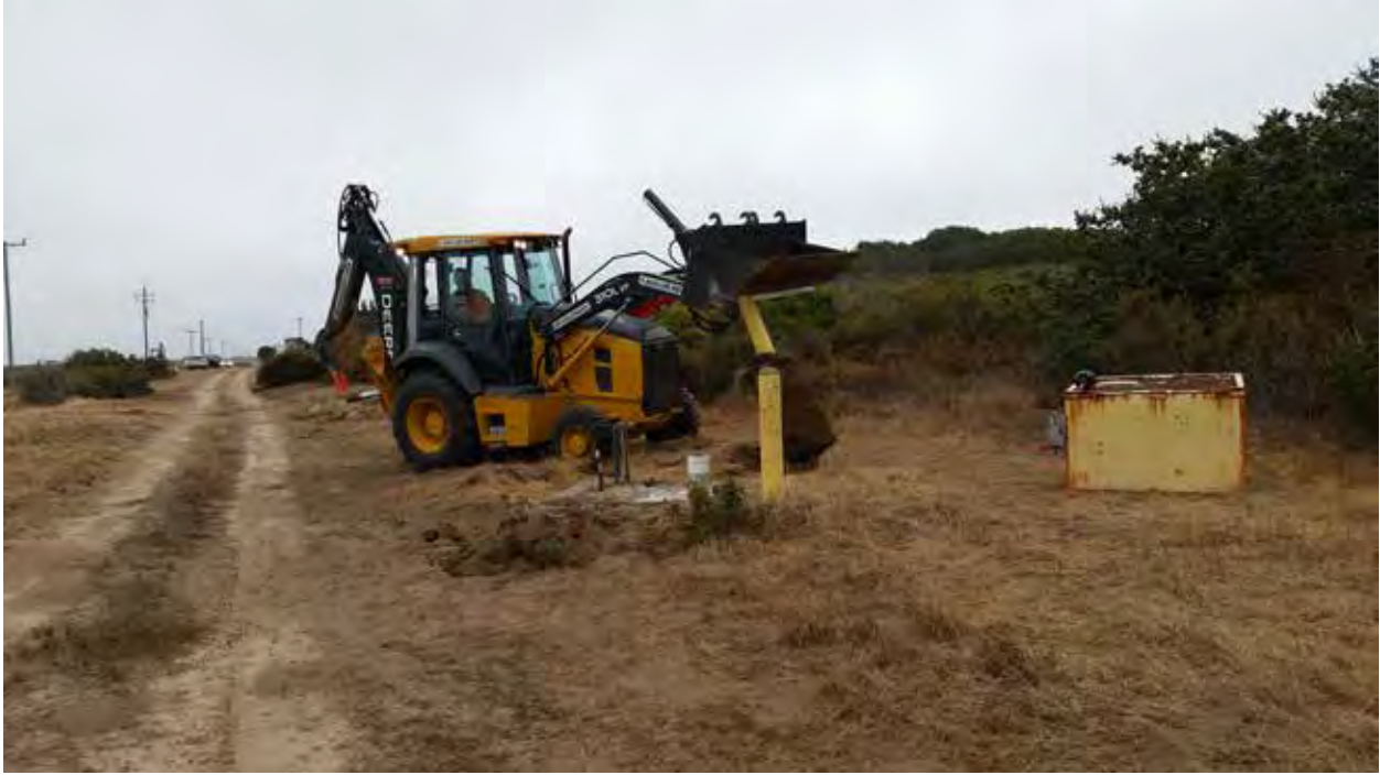
Removing bollards at well site on northwest boundary
