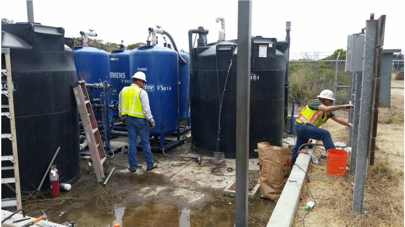
Photo 02 – Disassembling NWTS.
