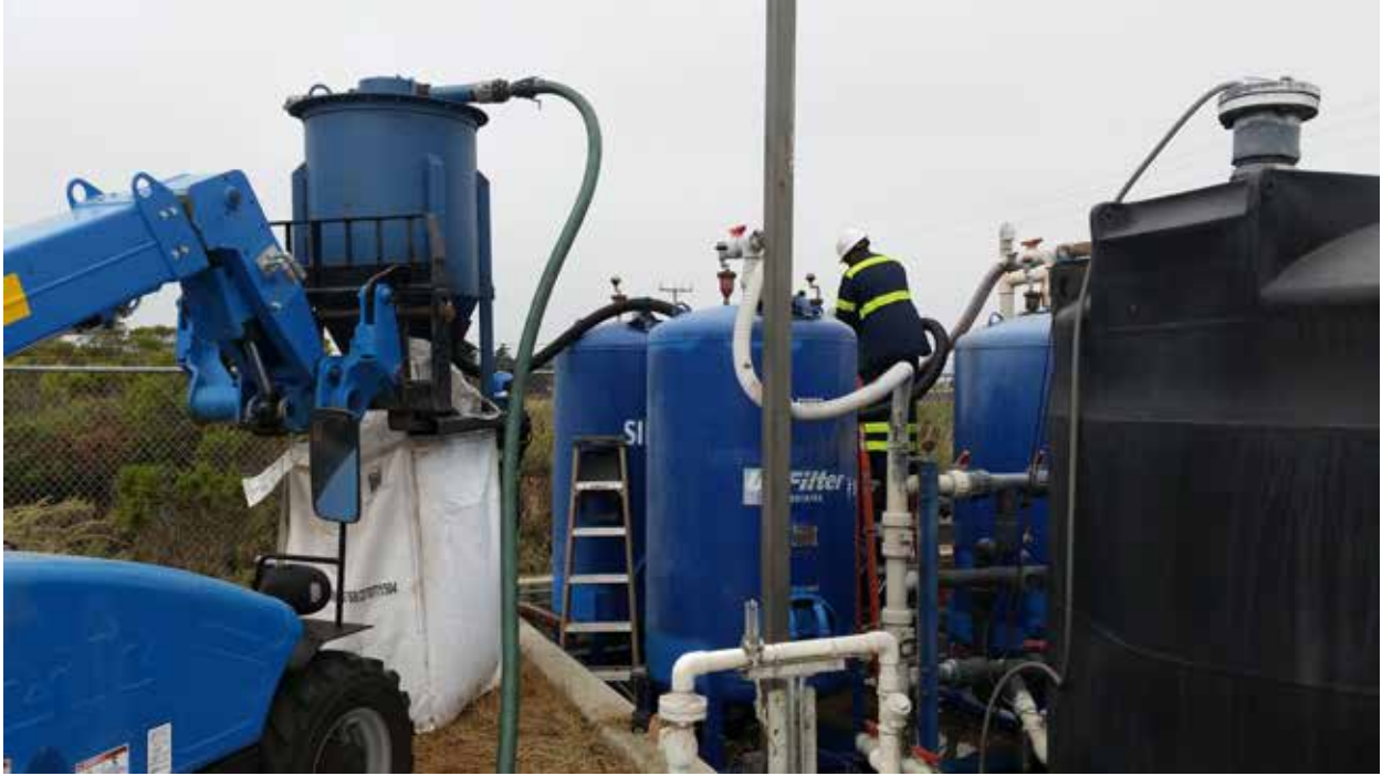
Removing carbon from NWTs treatment vessel
