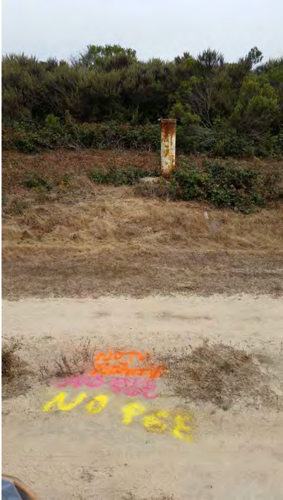
Utility clearance on northwest boundary road
