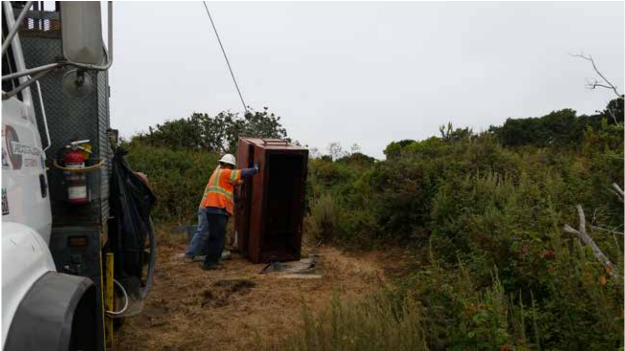
Removing JOBOX type well housing
