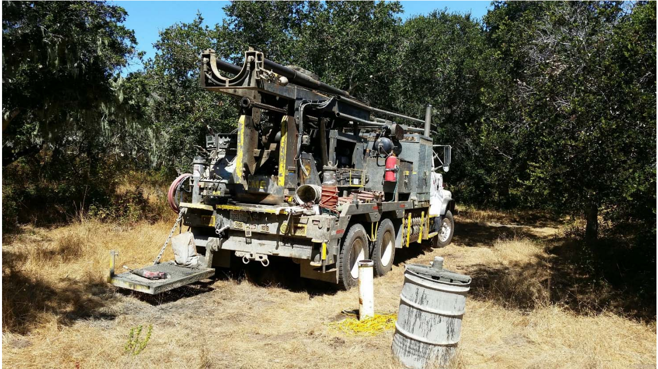
Photo 01 – Setting up to pressure grout.
