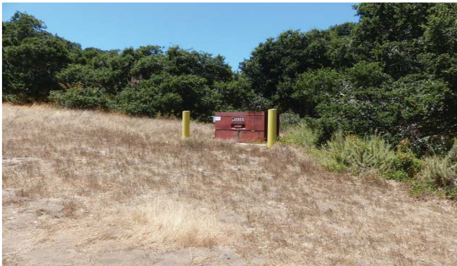
Photo 27. OU-1 FONR Well Site EW-OU1-71-A Prior to Destruction. (July 11, 2017)
