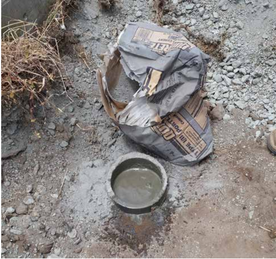
Infiltration trench pipe sealed with concrete
