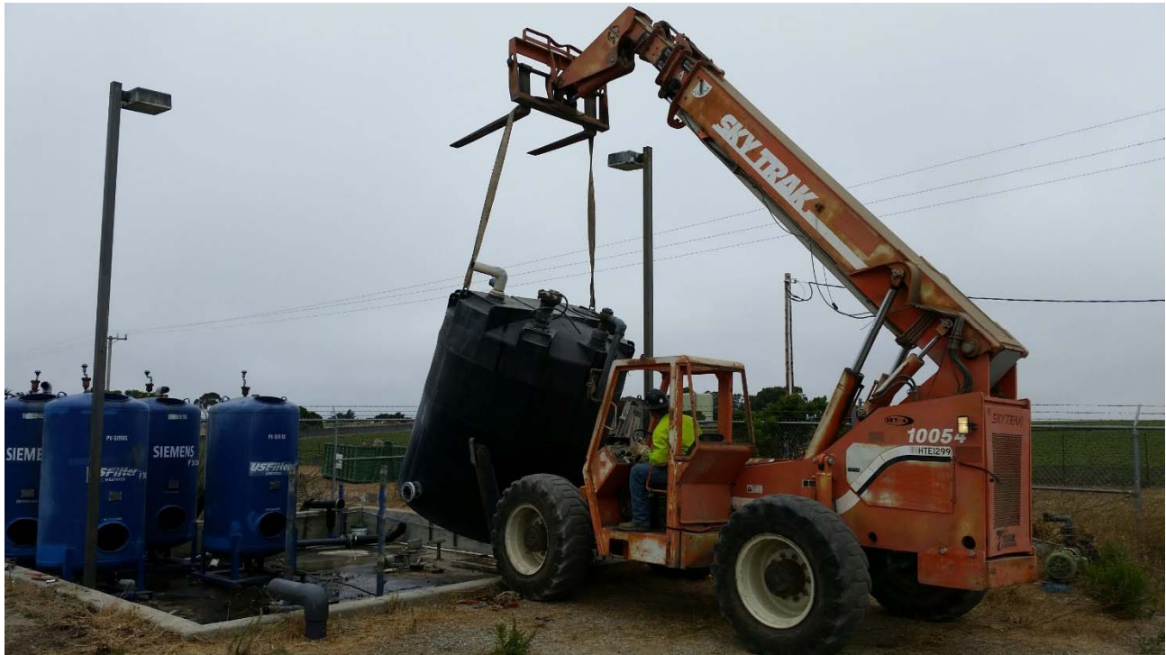
Photo 01 – Removing holding tank at NWTS.
