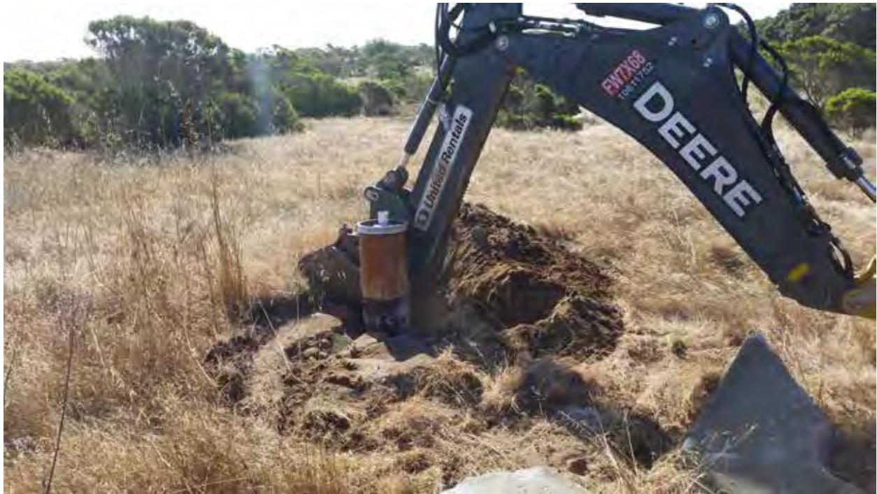
Removing well casing to 5 feet below ground
