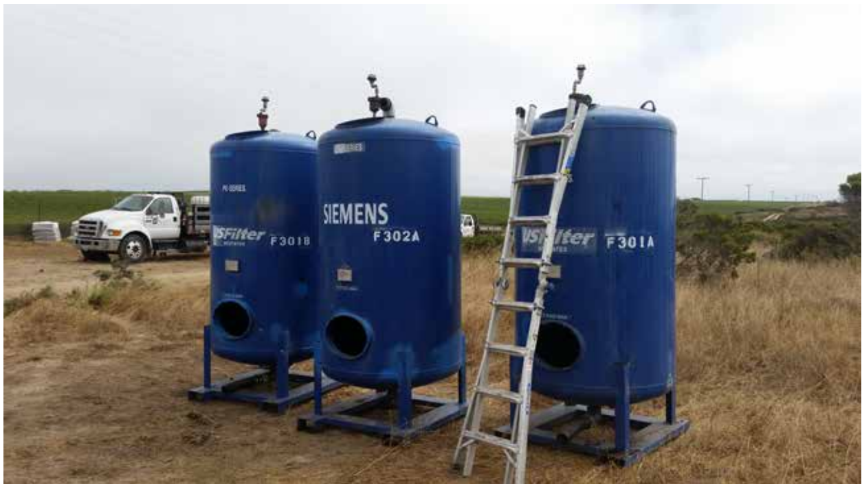
Remaining carbon vessels removed and staged for transport
