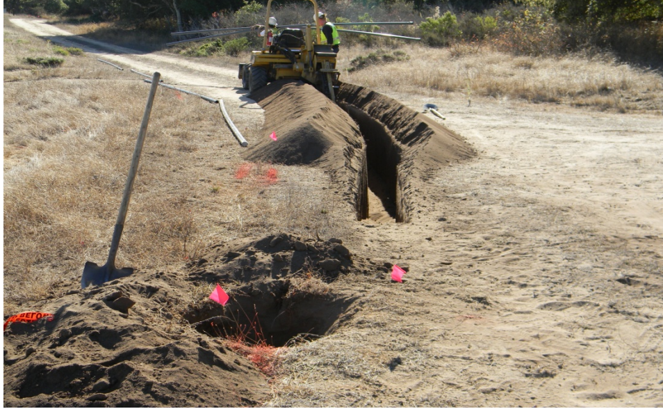
Photograph 1.1 – Typical Trench Construction
