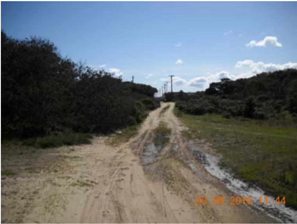
WCS# 1A ps84a Staging Area Pre-Treatment 09 March 2010
