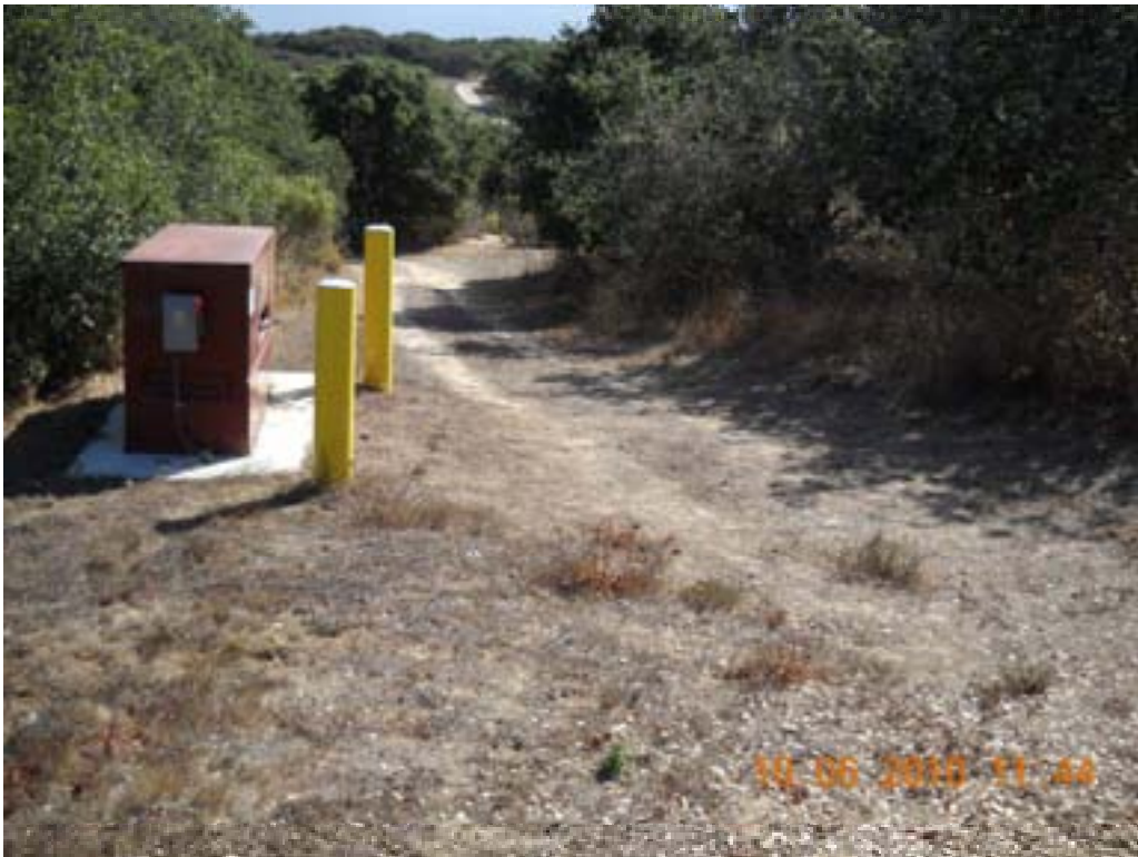
WCS# 12B ps48a MW-OU1-85-A Post-Treatment 6 October 2010
