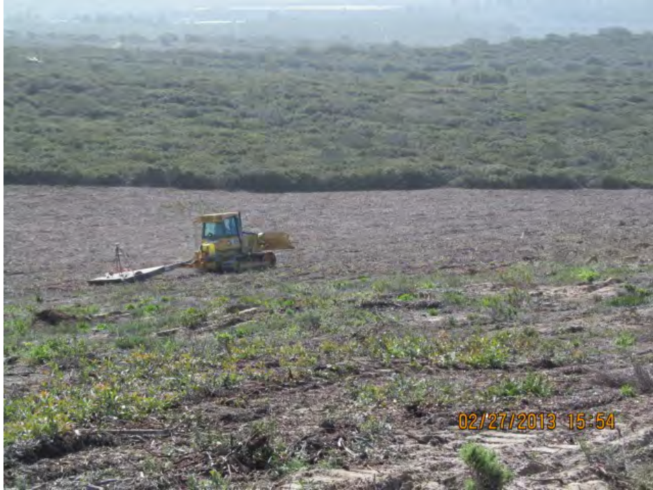
Photograph 5 - DGM Survey Operations – 1
