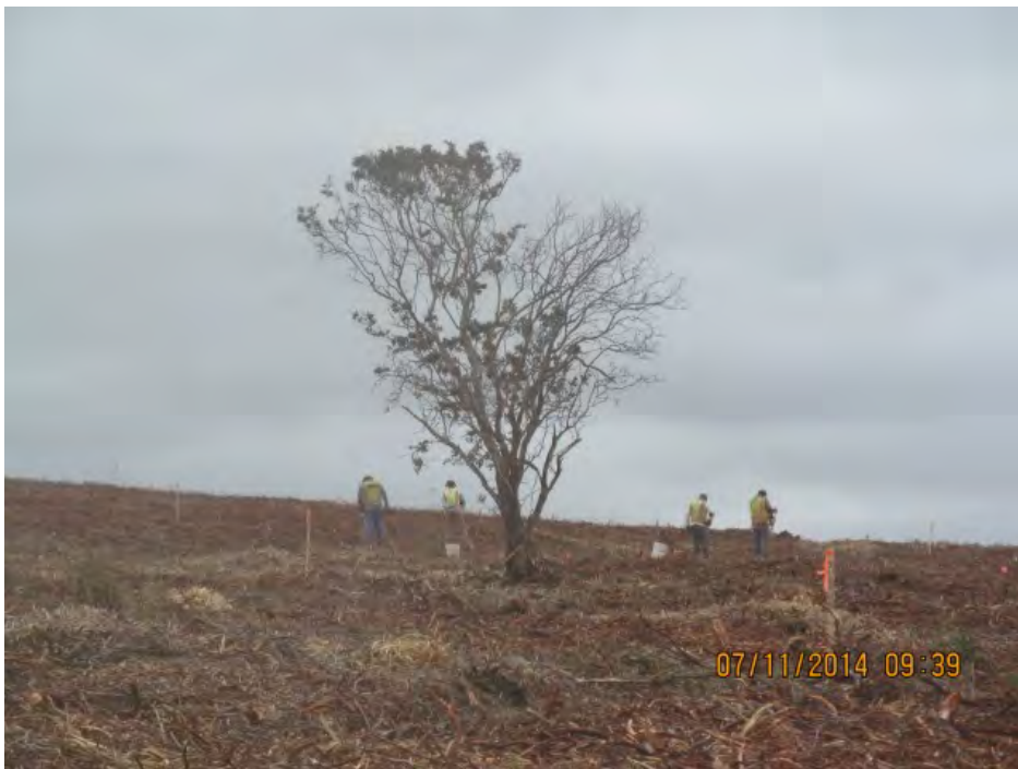
Photograph 4 – Surface Removal Operations – 2
