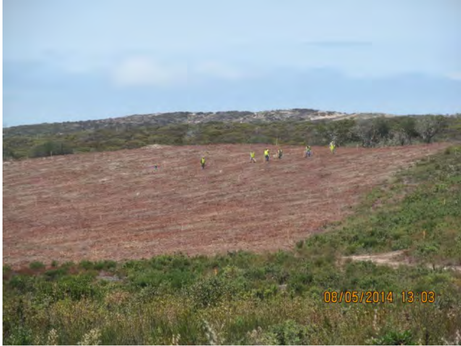
Photograph 3 – Surface Removal Operations - 1
