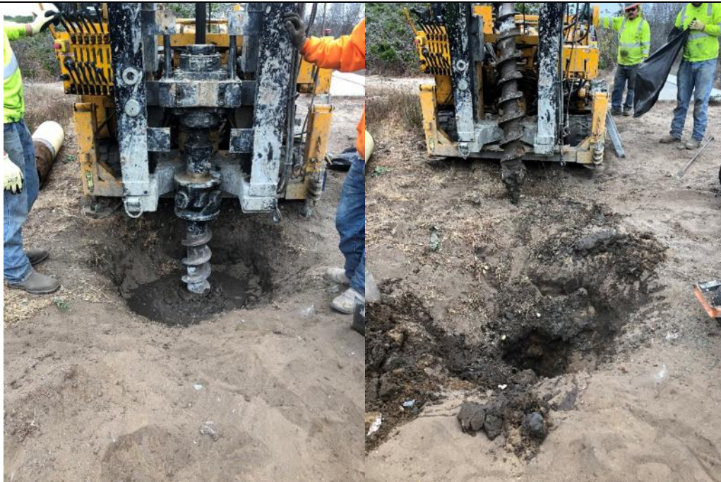
Description: Well casing is drilled down to 5' bgs.
