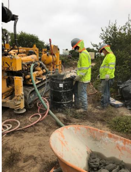
Description: 95% Portland Cement / 5% Bentonite is mixed at MW-BW-69-A.
