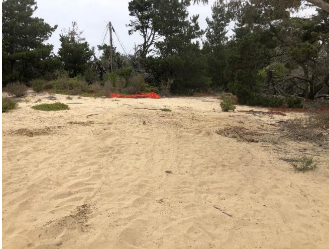
Description: MW-OU2-33-A after Well Decommissioning.
