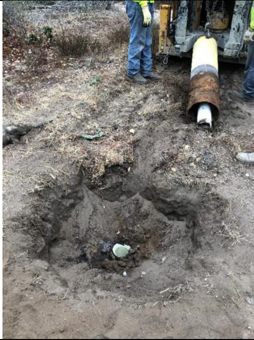
Description: Well casing is cut at MW-BW-22-180.
