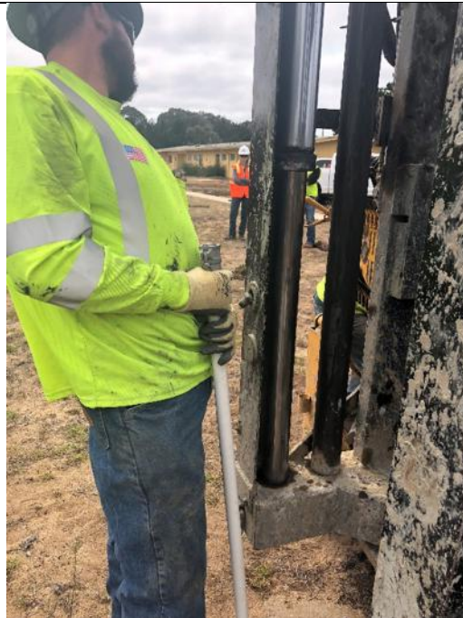
Description: Installation of the tremie pipe at MW-OU2-36-A.
