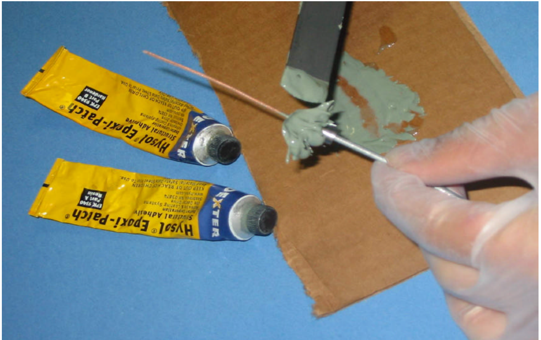
Pic.15 Apply epoxy. Cover the trimmed armor strands with epoxy
